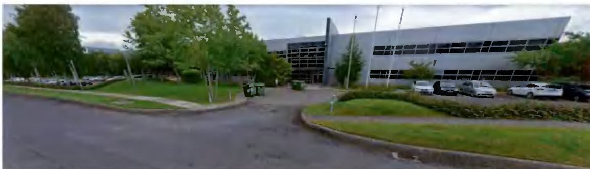
Figure 3: front (west) elevation view of the site
