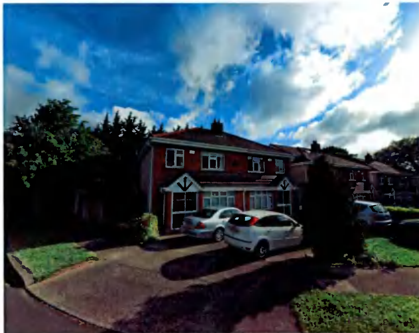
Fig. 7 Semi-detached houses immediately south of site, looking NE from Grangebrook Ave
