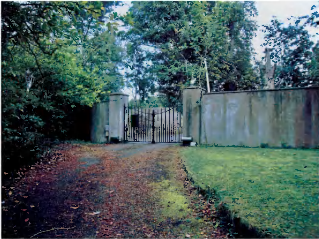
35 Southern gate looking out towards main roadway
