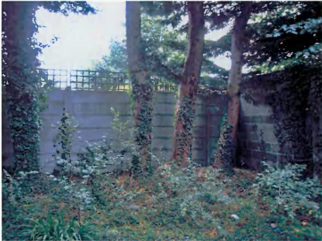
15 Junction of south boundary with west boundary wall along Grangebrook Avenue
