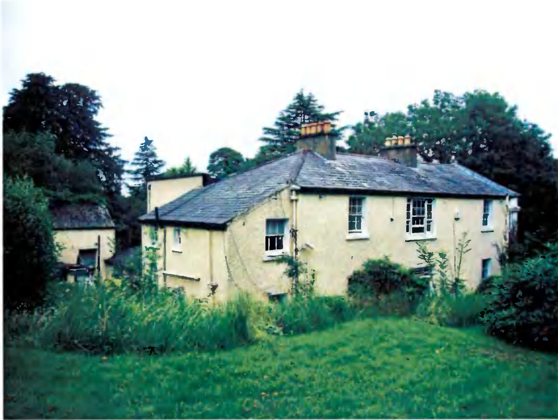
3 Southern facade and rear seen from upper garden
