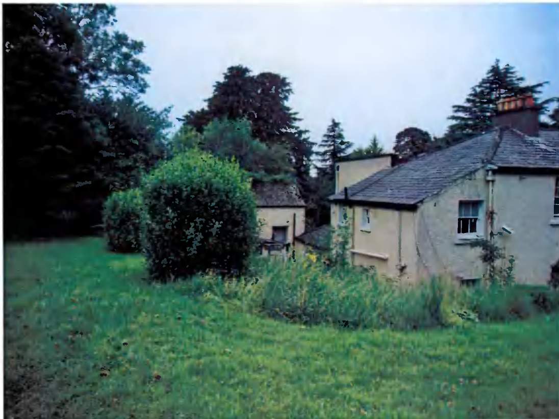
6 Upper garden and rear of house looking northwards
