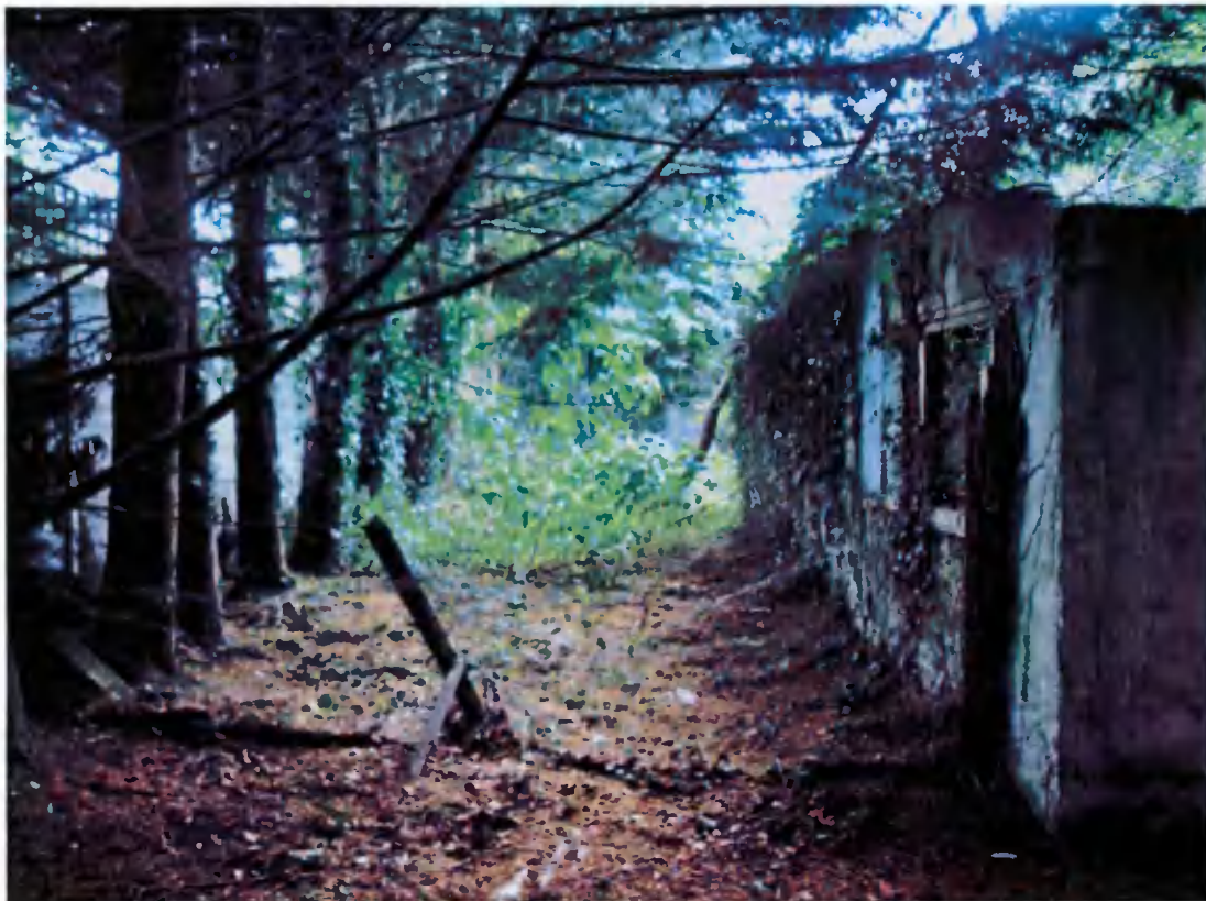
14 Looking west along boundary wall
