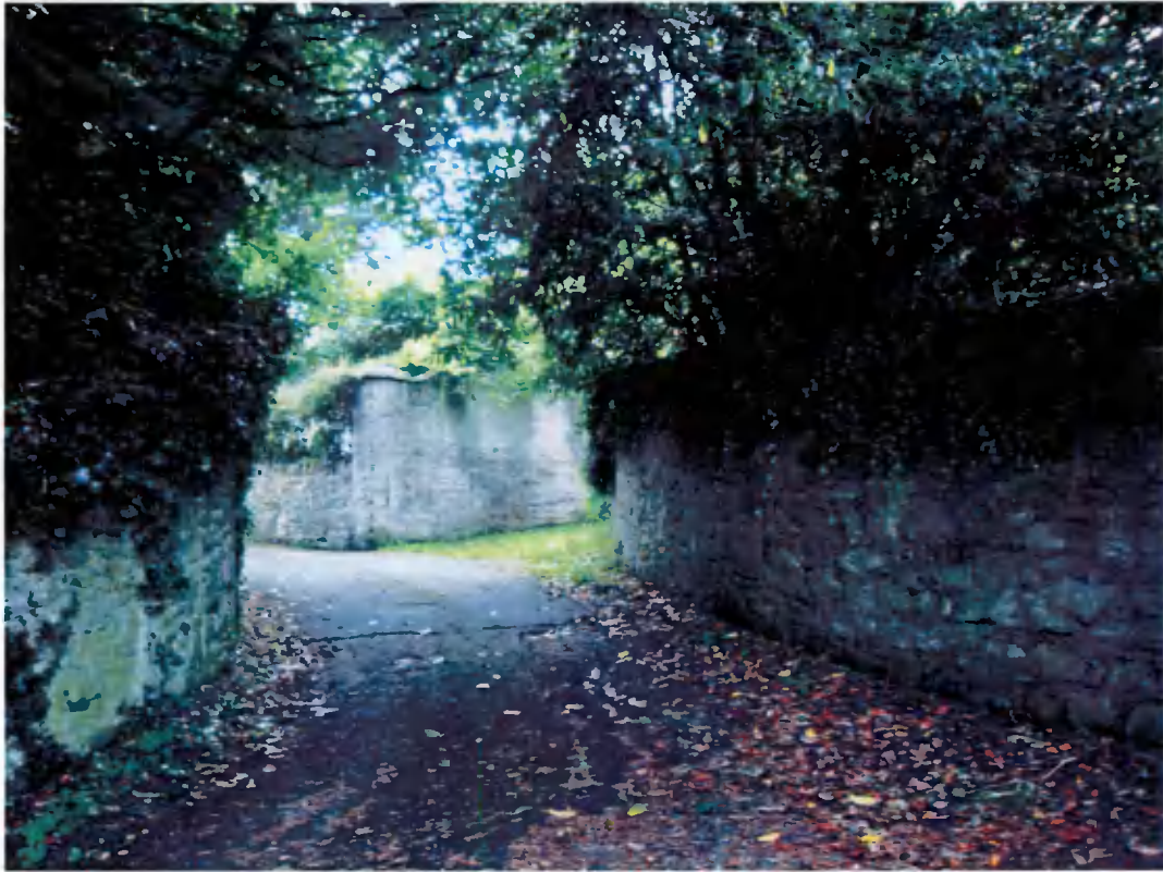
27 Lane at curve to Palmyra entrance gate, wall of Whitechurch on right, looking SW
