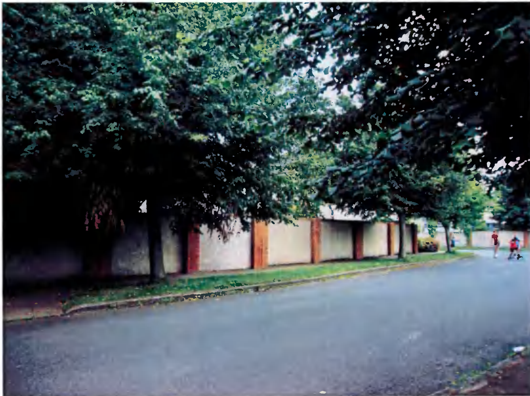
38 Modern wall towards the southern end of the western boundary
