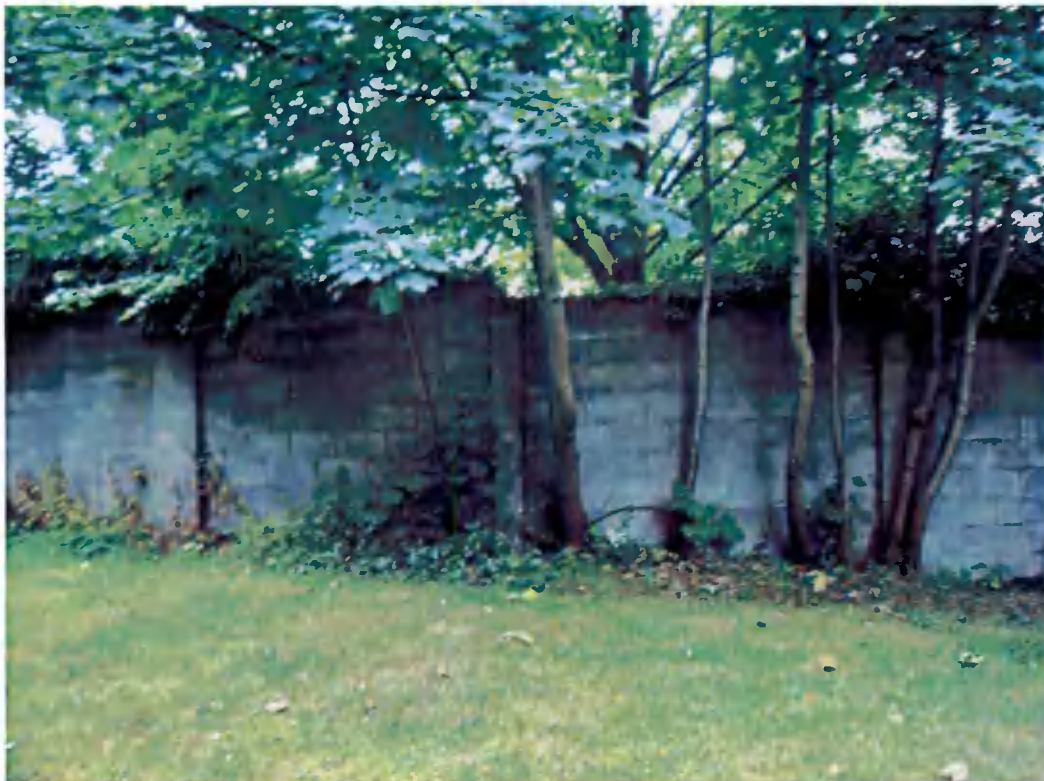
20 Eastern face of boundary to Grangebrook Avenue
