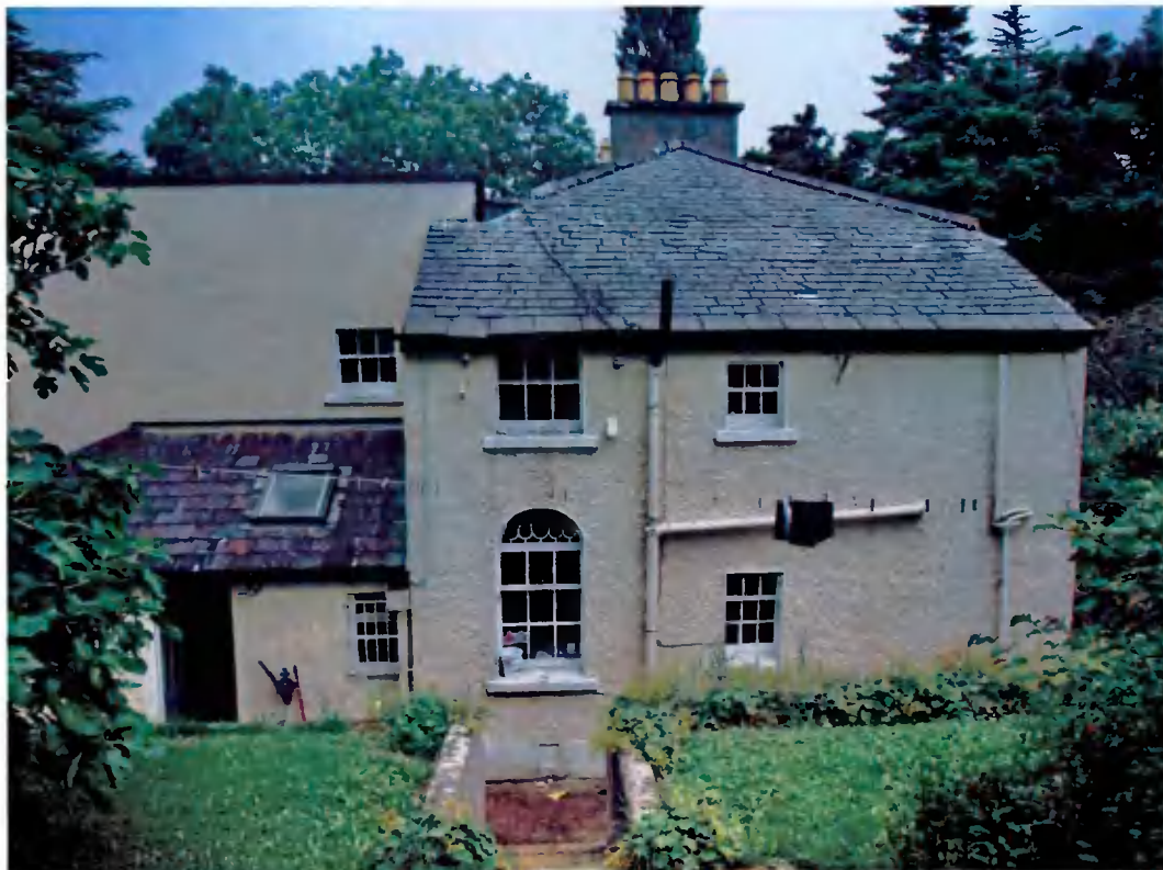
2 Rear, western, facade
