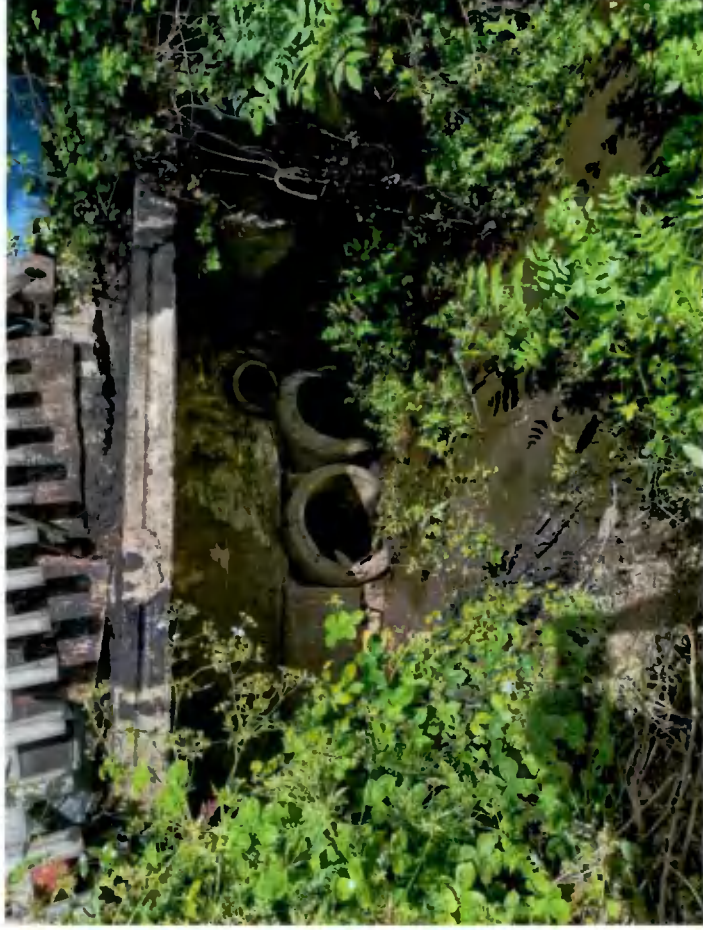
Figure 5-4 Inlet to culvert at downstream boundary
