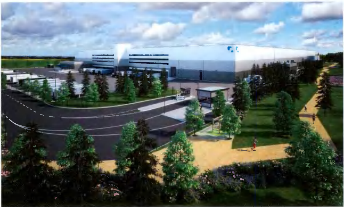
Fig13: Indicative CGI of riparian parkland setting to west and south of Units E, D & C
