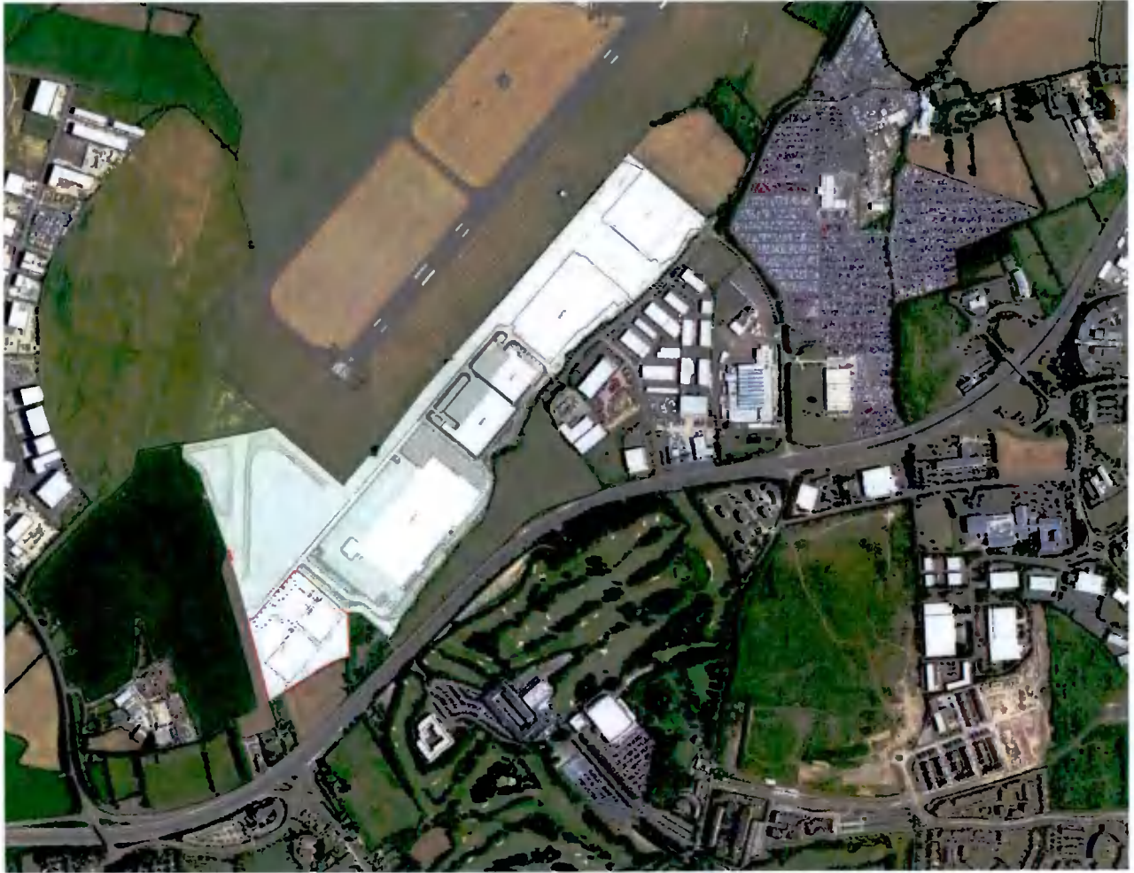
GOOGLE VIEW - MOUNTPARK BALDONNELL PHASE 1 & 2 AND ADJOINING LANDS
