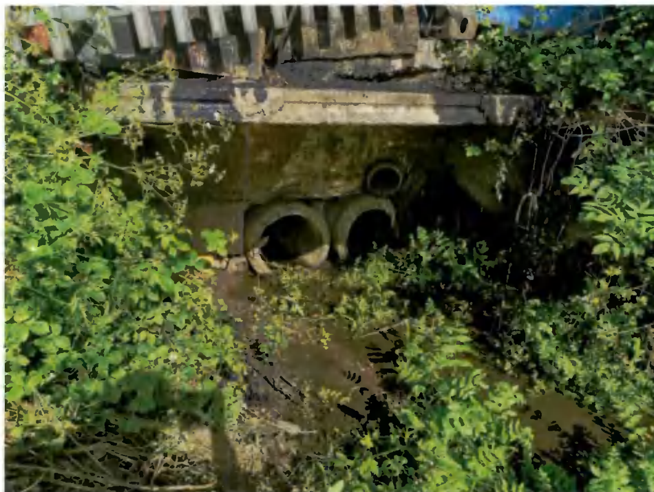
Figure 5-4 Inlet to culvert at downstream boundary
