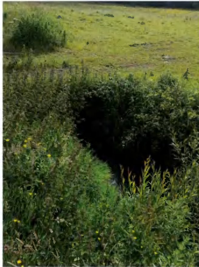
Figure 5-5 Inlet to culvert midway through the Site
