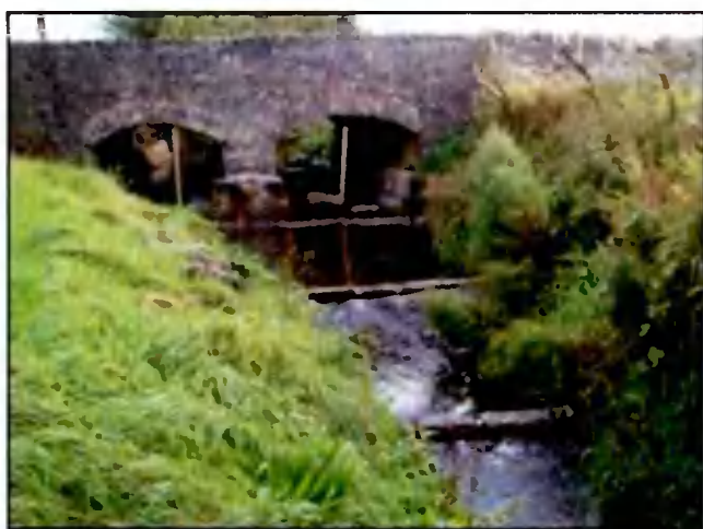
Low level stone weirs installed on a salmonid nursery stream to back water the bridge apron /scour slab originally installed at too high a level.
