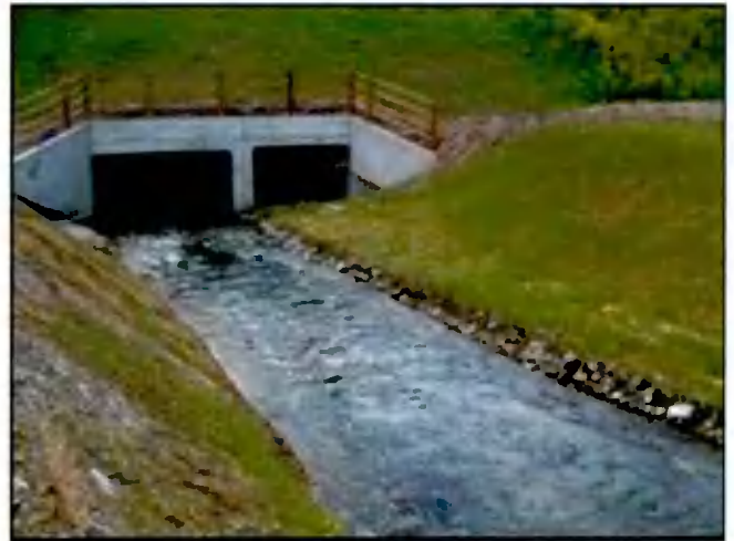
Looking from upstream towards a culvert arrangement. Moderate and flood flows are conveyed in the right hand culvert. Entry to that culvert is dictated by the invert and contour of the right hand portion of the newly created river channel. The left hand bank finished batter angle is approx. 45°. The first portion of the right hand bank to convey the moderate flow is battered to approx. 30°. The extreme right bank area is battered to approx. 45° to convey flood flows.
