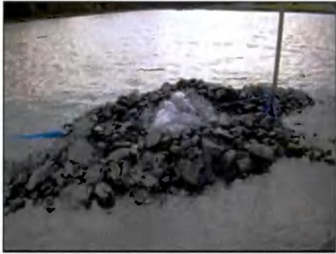
Silt control pond. The blue hose conveying pumped silt laden waters has its outlet securely anchored within the stone aggregate thereby dissipating energy, minimising disturbance, and preventing pond contents being disturbed and re-suspended.
