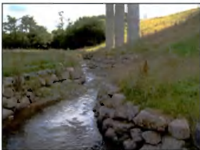
Suitably sized rock armour built to high water level at a location influenced by tidal back-up.
