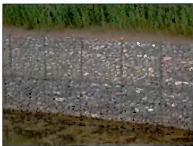
Visually unsightly stone filled gabion baskets.
