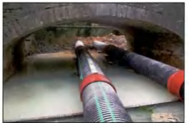
Repairs to a single arch bridge and scour slab with stream flow piped from upstream to downstream (foreground) during both grouting and slab repair.
