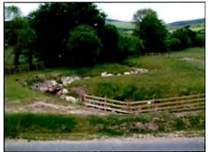
Extreme meanders installed during excavation of a new channel to overcome excessive gradient between the original course of the stream (in the background at tree line) and the point of entry of the newly created channel to a culvert (in foreground under the timber fencing). In this instance there was inadequate provision at the planning and design stage for the necessary land take.
