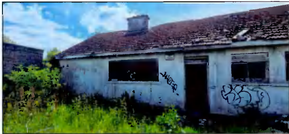
Front elevation of abandoned dwelling
