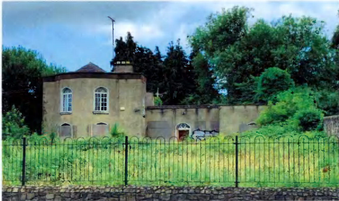
North (front) façade of Newbrook House from Taylor's Lane
