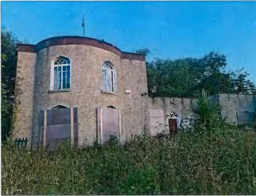
Plate 1. View of the front of Newbrook House
