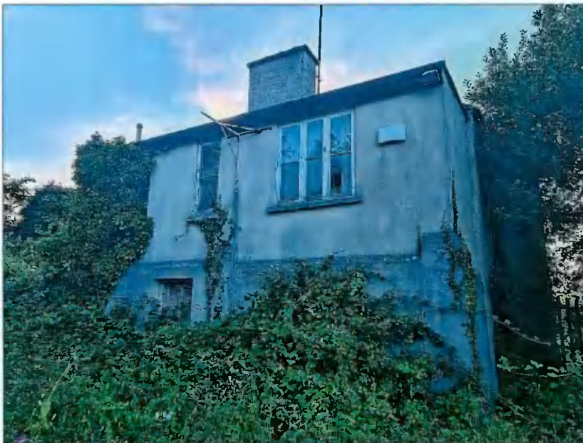
Plate 2. Rear view of Newbrook House
