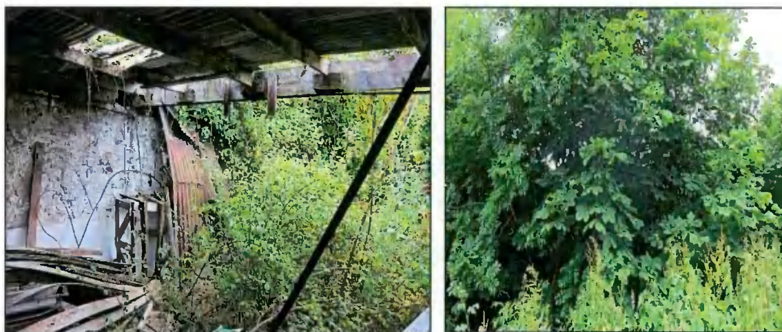
Figure 5.3.2 Disused Outbuildings and Immature trees with low to negligible potential for bat roosting
