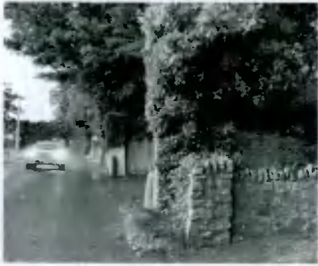
Stone wall and fence
