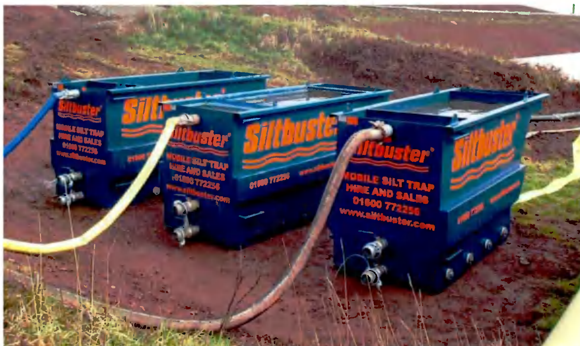
Figure 5-3 Temporary site settlement tanks (Source: Siltbuster)
