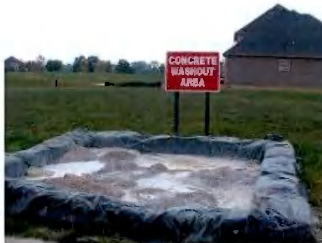
Figure 5-4 Example of temporary concrete washout area
