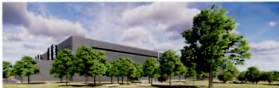
Picture 41: View from south east position showing data halls & screen enclosures to generator yards
