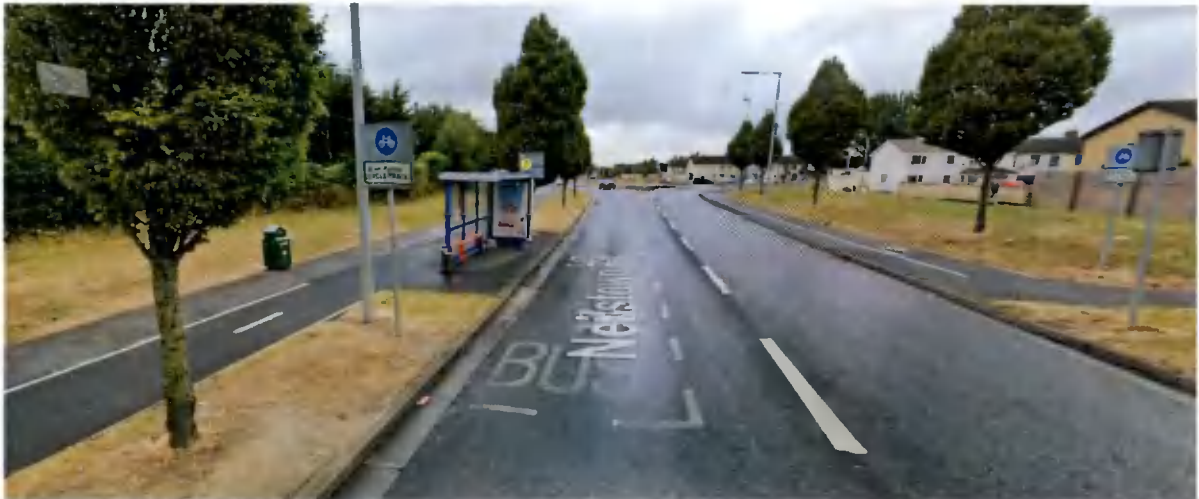
Figure 1.2 – Cycle tracks on Neilstown Road
