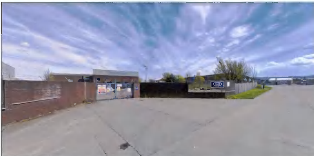
Figure 1.3 Street view of the existing entrance to the site accessed from Ballymount Road Lower (source: Google Maps, cropped and annotated by Tom Phillips + Associates.)
