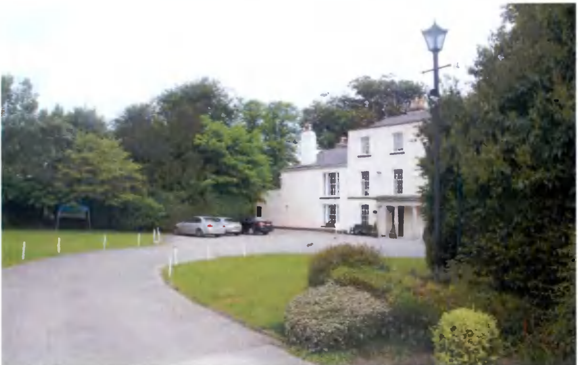
Fig. 12: Sally park house approach from entrance.
