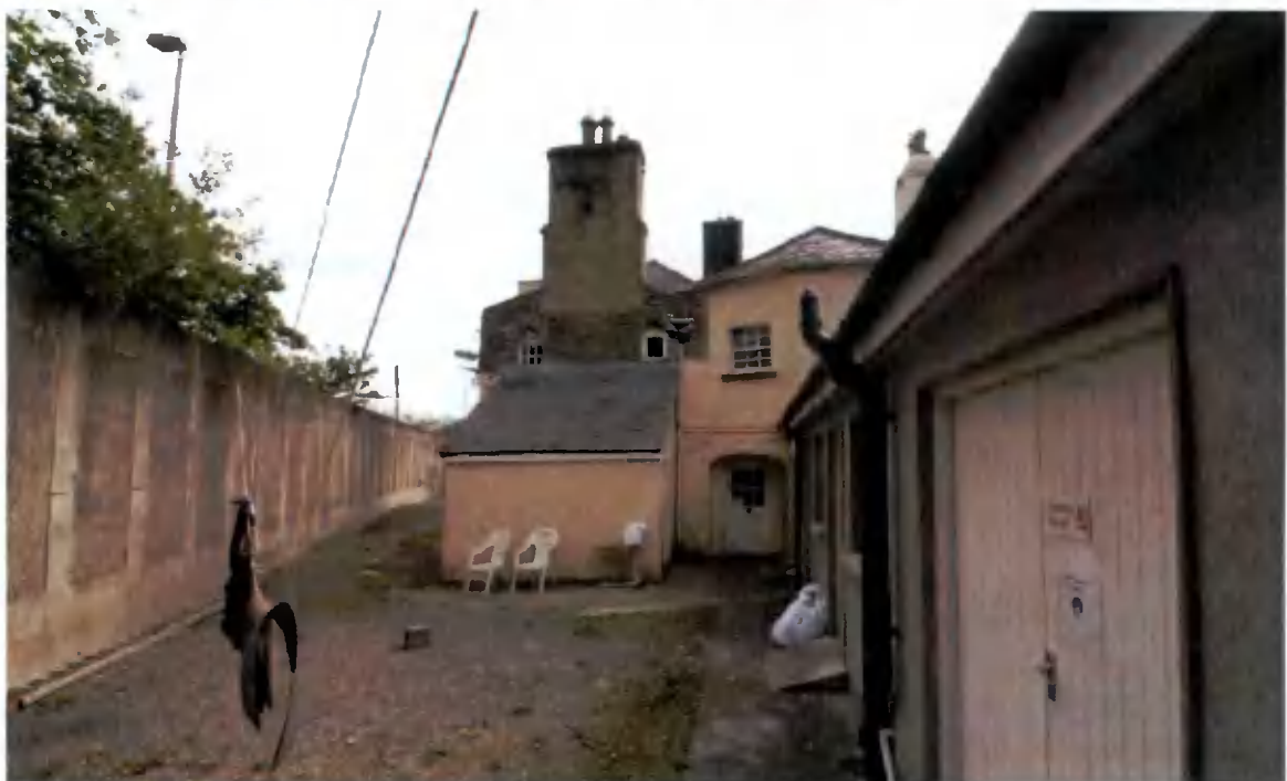
Fig 29 & 30. Rear yard existing to West.
