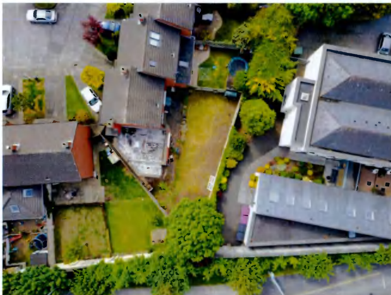
Fig 35. Eastern end of site.
