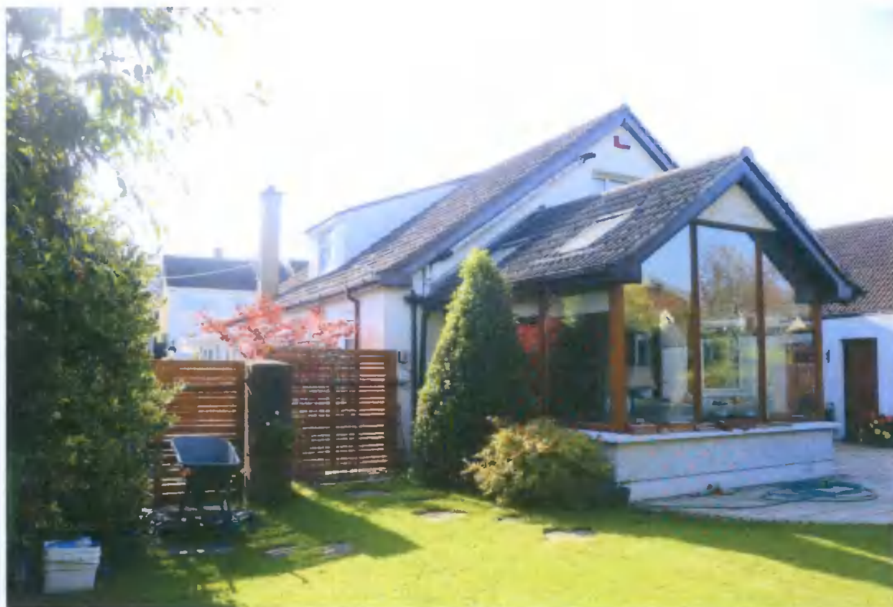
Image 6.2 Eastern elevation of Fitzgerald property that will be affected by proposed 4 storey building
