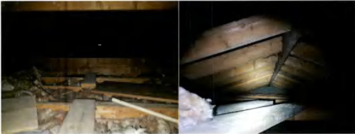
Plate 3-7 & Plate 3-8: Attic space.
