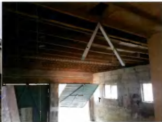
Plate 3-10: Internal view of shed
