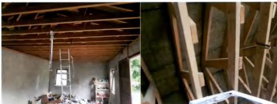
Plate 3-15 & Plate 3-16: Internal view of shed.
