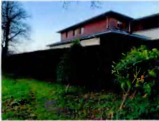
Existing boundary with 2m high railing & hedge around Rookwood View.
