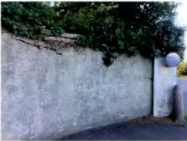
Wing wall and outer gate pier.
