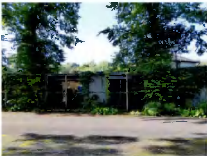
Existing garage to be demolished to create new entrance in wing wall in location of original historic courtyard entrance.
