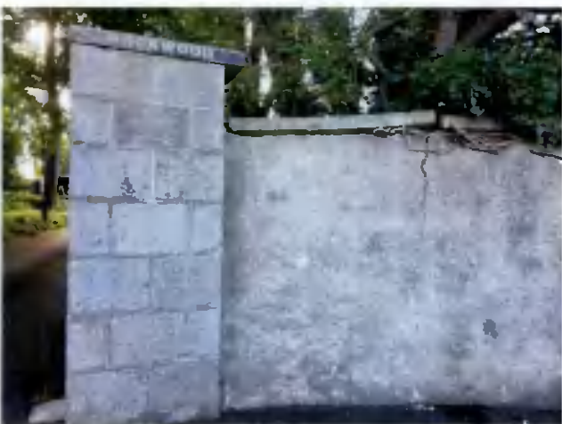
Inner gate pier and wing wall to right of entrance.
