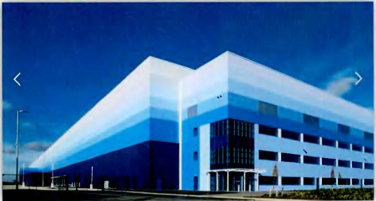
Figure 8.2: Altitude building with 21 m clear internal height in Gallagher Logistics Park at Magna Park, Milton Keynes, UK
