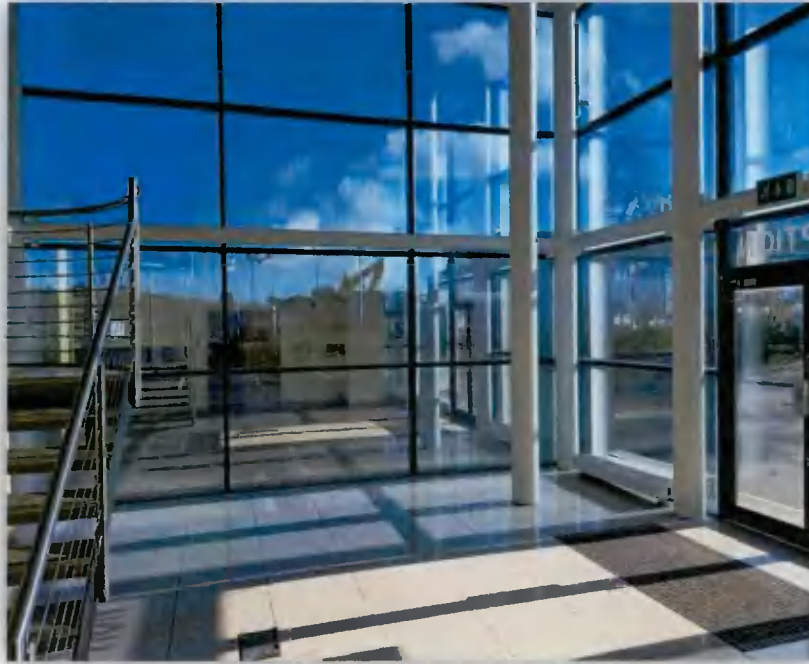
Figure 8.4: Internal view on Curtain walling
