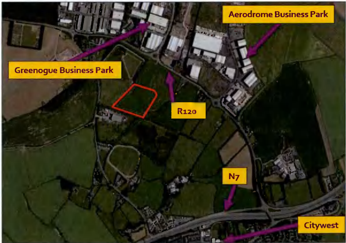
Figure 2.2: Aerial View of the Subject Site as Shown in Red (Indicative Only).
