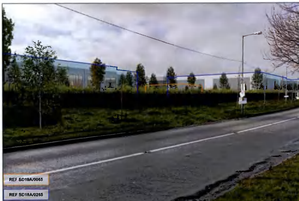
Figure 5.4: Image Showing the Now Proposed Development and Neighbouring Development Permitted Under SDCC Reg. Ref. SD18A/0265 and SD19 A/0065 from College Lane.
