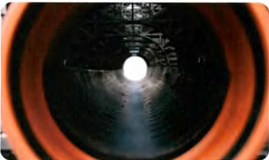
Connection to low flow maintenance channel at invert level.
