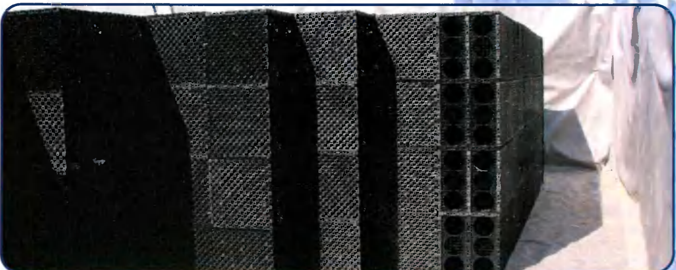
Tank 2mts deep with access channels.
