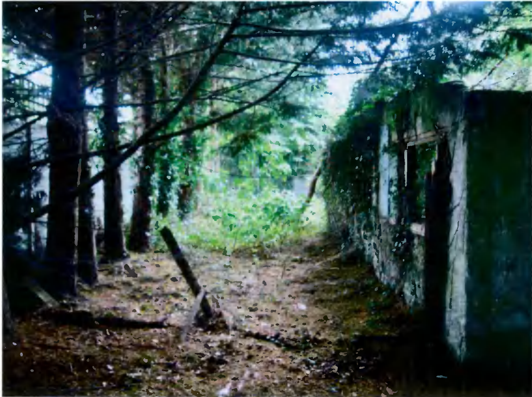
14 Looking west along boundary wall
