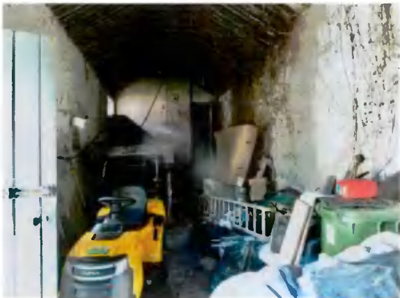
85 Interior of garage looking west
