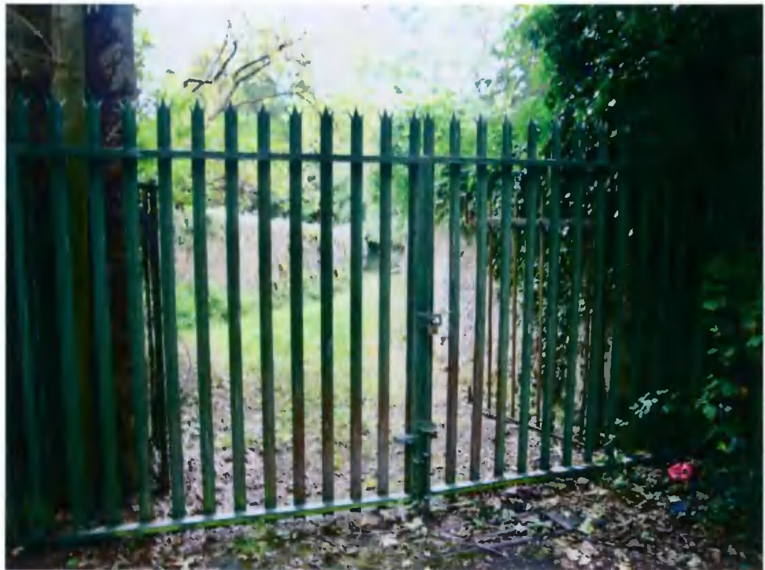
24 Gate in site boundary, looking eastwards to lane which has Whitechurch wall on left
