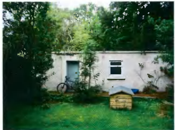
93 Southern end of sheds
