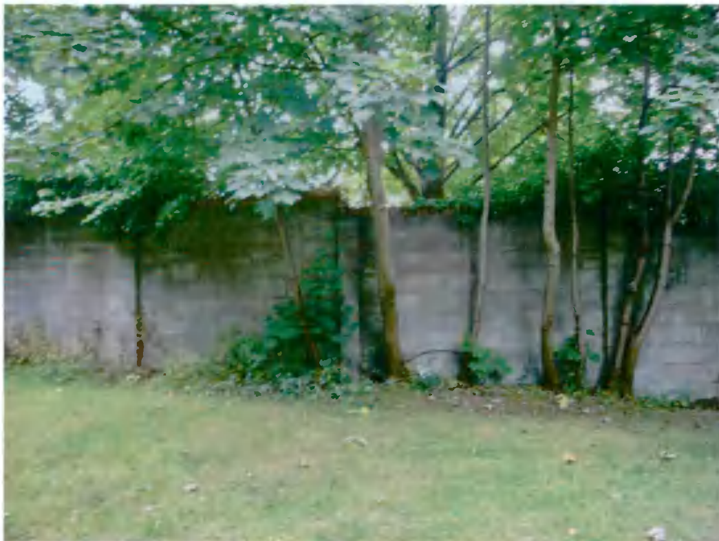
20 Eastern face of boundary to Grangebrook Avenue
