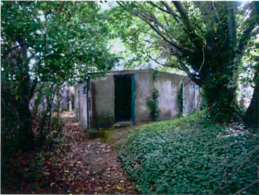
12 Modern shed in south-west corner of site
