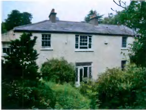
77 Rear west facing wall
