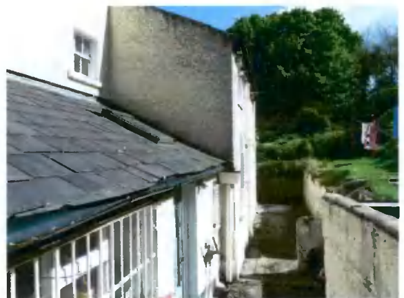
82 Lean-to extensions on west facade, looking south-east
