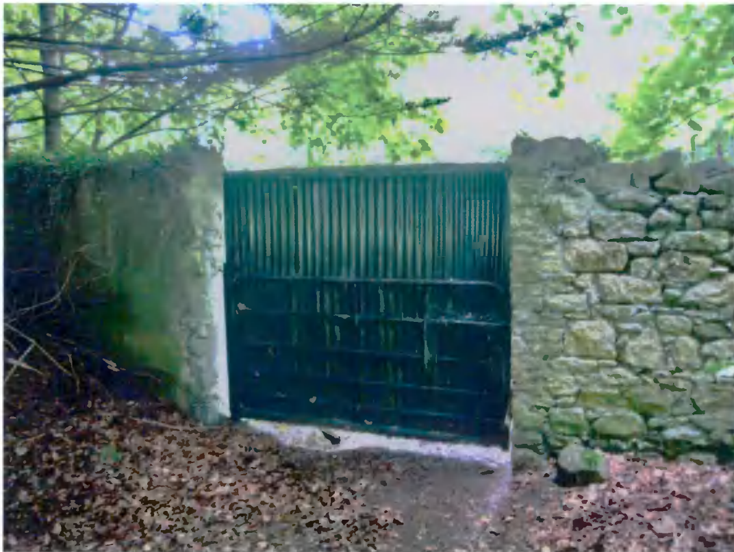
16 Gate in stone wall running east -west across site, seen from south
