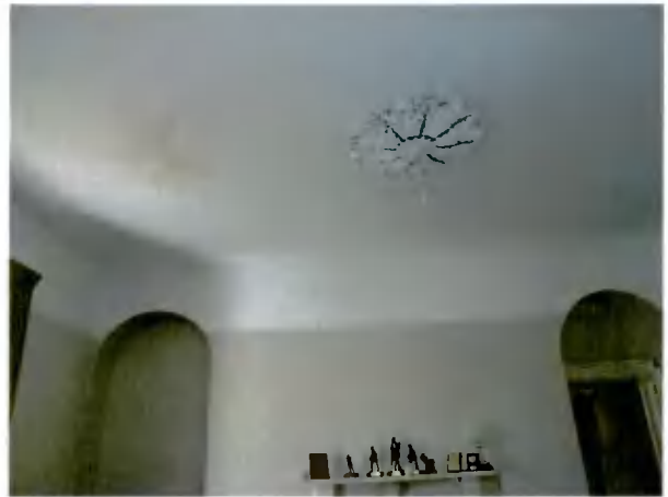
10 Living room 1 ceiling
