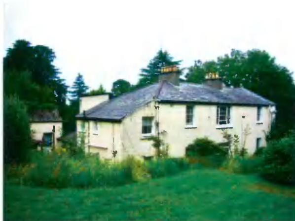
79 South and west walls, and detached garage on left
