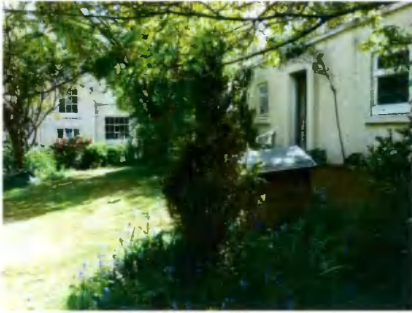
95 East wall of sheds, looking south to north wall of house
