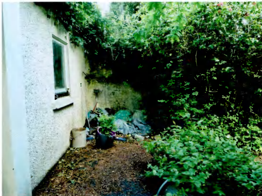
Fig. 27 Existing Garden Shed 1. Junction with boundary wall to Lane. Looking north-wards
