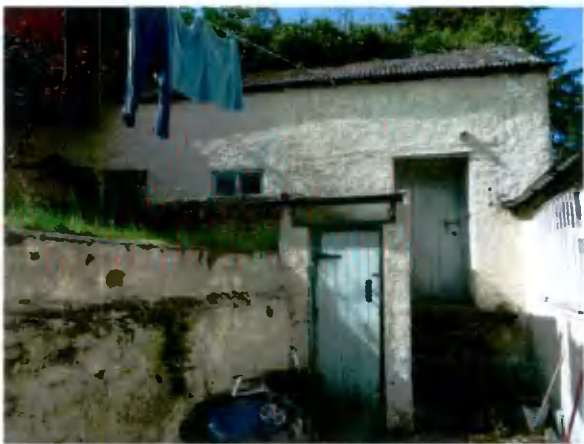
84 Walls, shed and garage
