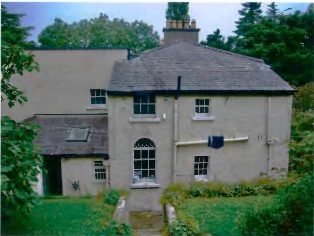
2 Rear, western, facade
