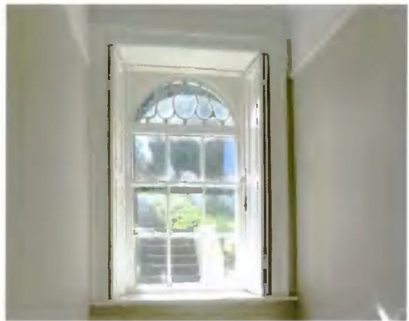
22 Window in SW wall of corridor. To be re-located to Stairs
