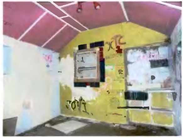
86 Rear room at west end of garage
