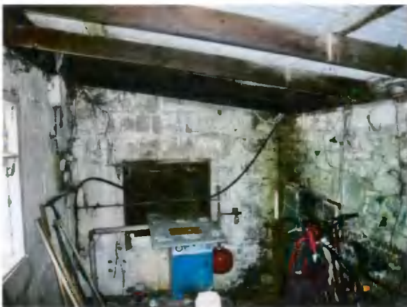
97 Interior of southern shed, looking south
