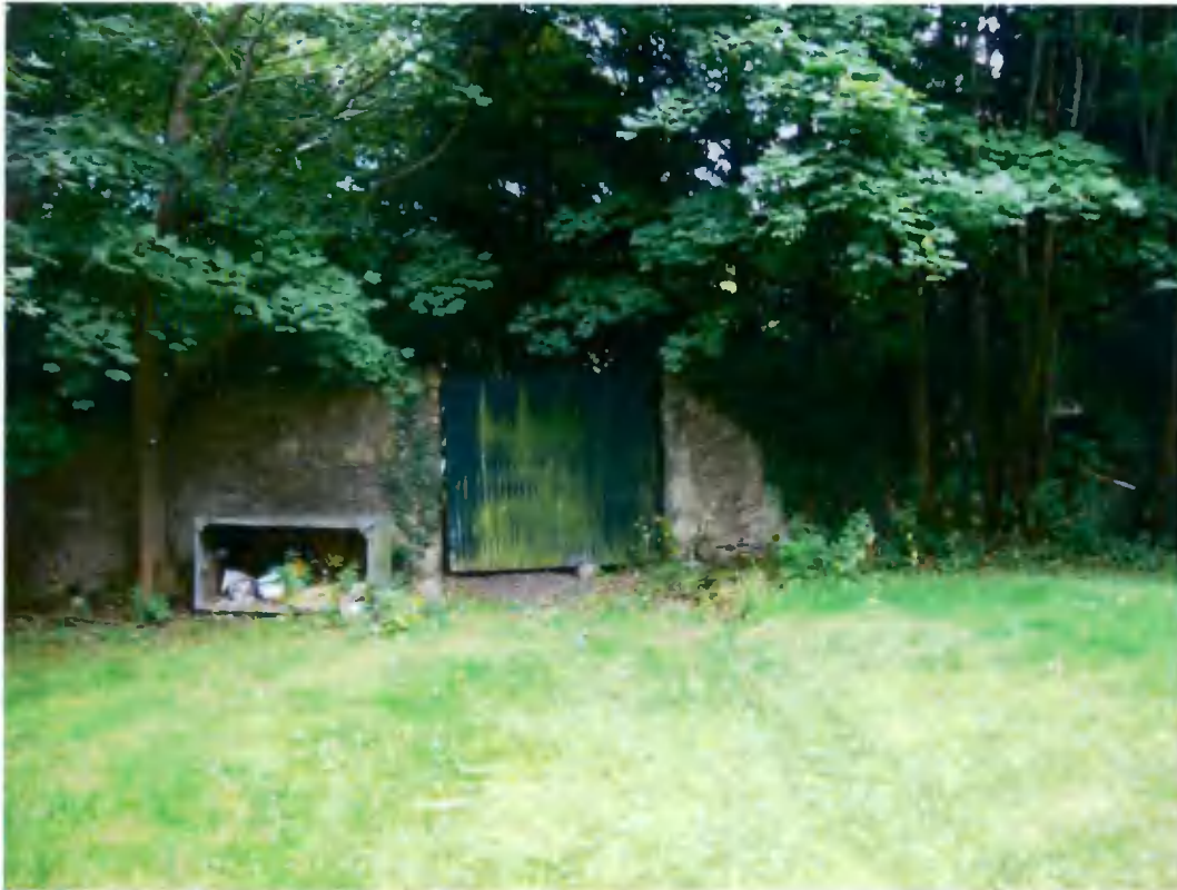
17 Gate in stone wall running east -west across site, seen from north
