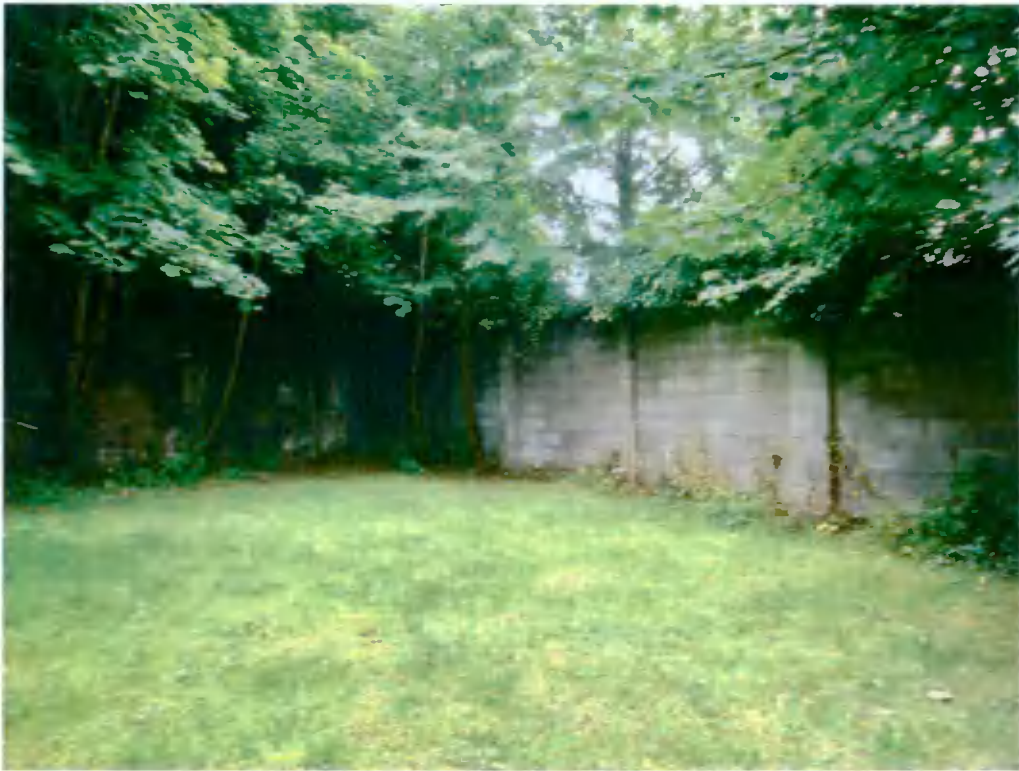
19 Grangerbrook Ave. block boundary running north from junction with on-site stone wall
