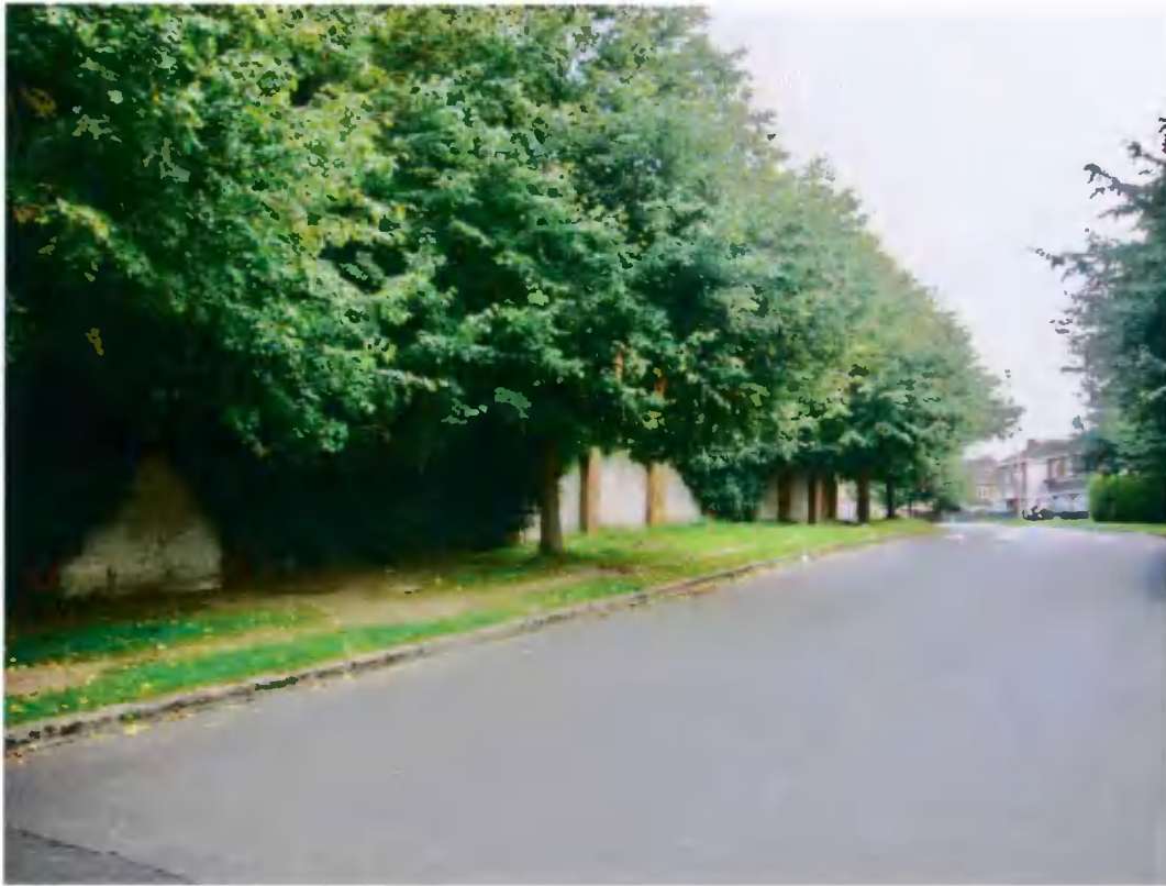
37 Looking south along western boundary wall of site at Grangebrook Avenue
