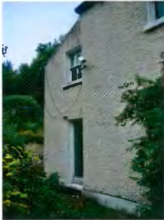
78 South-western corner seen from south
