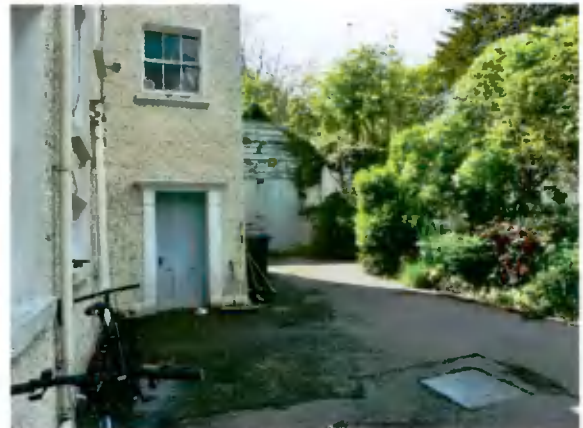
88 Kitchen entrance, garage and outhouses to left
