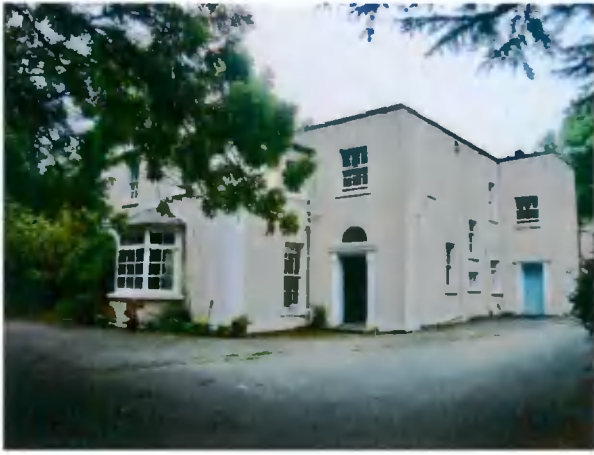
71 East and north facades
