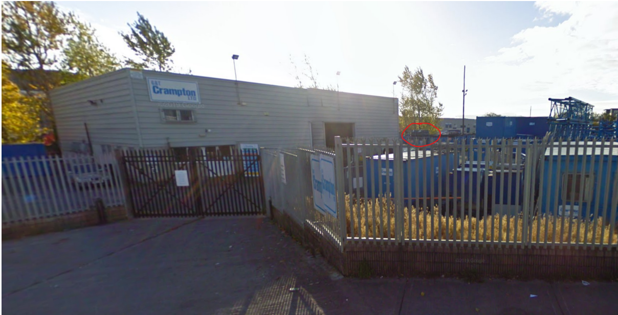
Street view of site in October 2010. Note oil tanks circled in red
