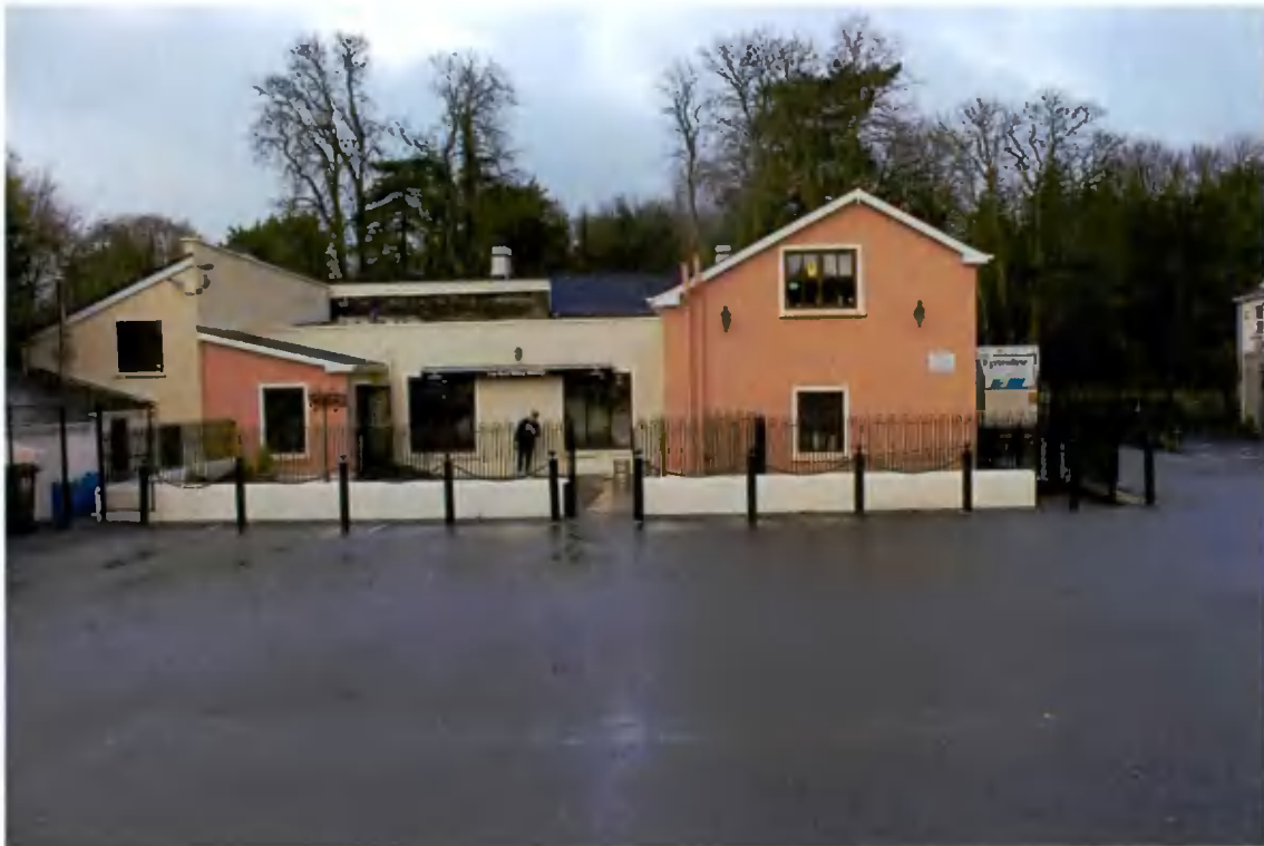
Figure 4: Rear elevation of Ball Alley House. (0615)
