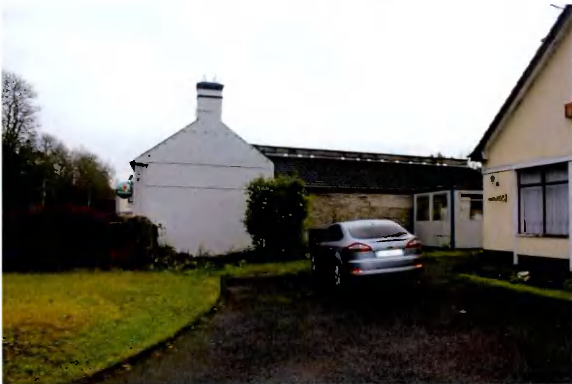
Plate 4: West gable of Ball Alley House. (0623)
