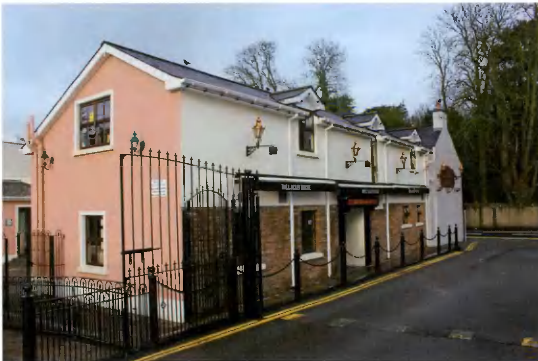
Figure 2: A later modern extension to the rear (southeast corner) of the building (0615)
