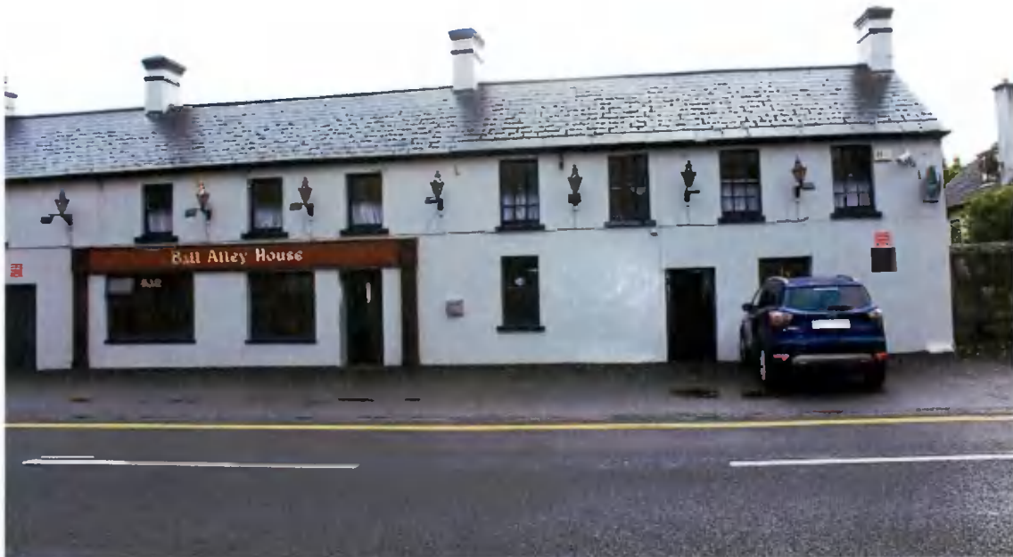
Plate 1: Early photograph of Ball Alley House façade west end. (0618)
