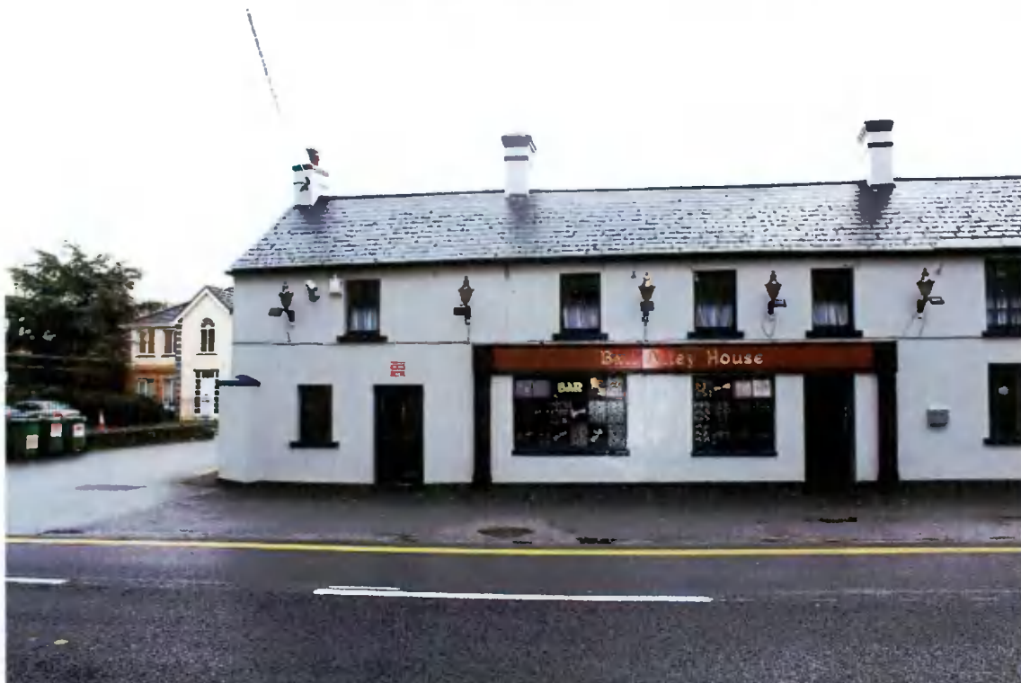
Plate 2: Early photograph of Ball Alley House façade east end. (0619)
