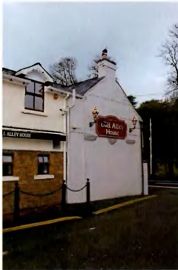
Plate 3: East gable of Ball Alley House. (0614)
