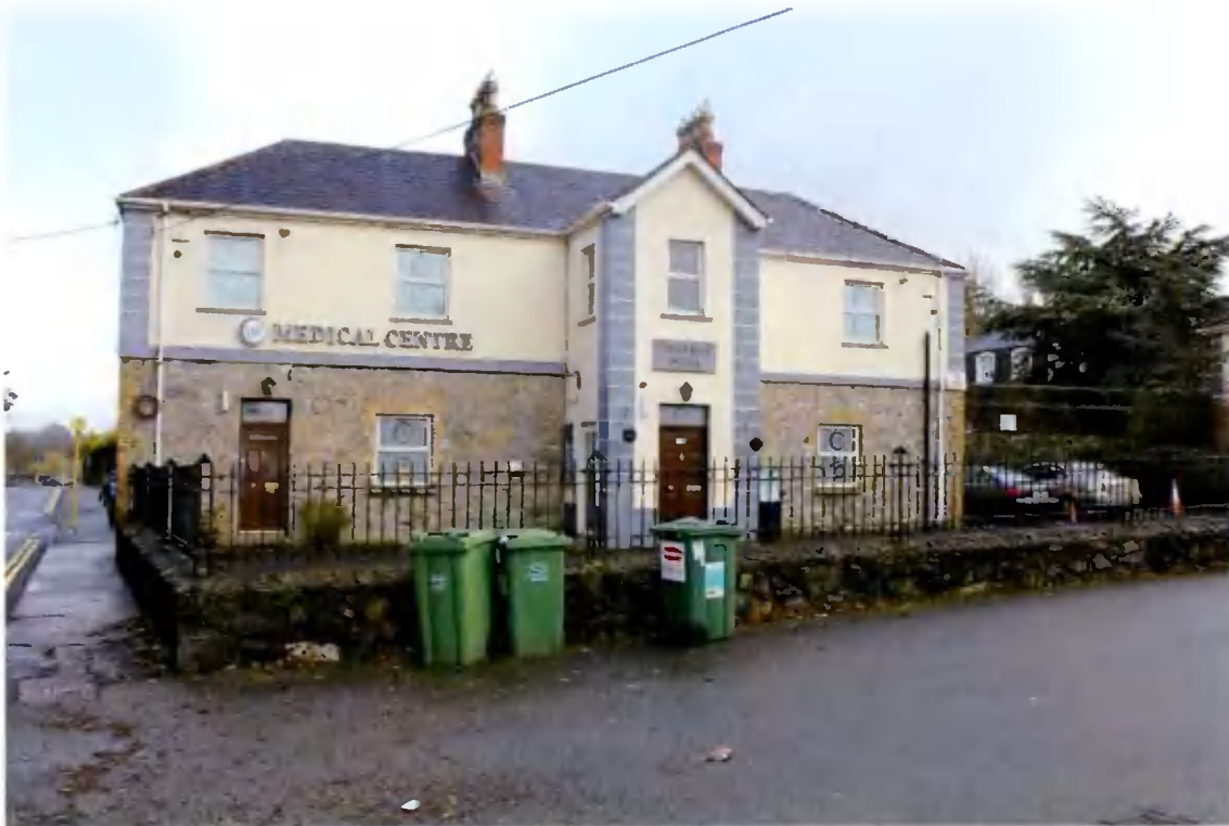
Figure 3: Side elevation of Ardfield House, which is to the east of Ball Alley House. (0615)
