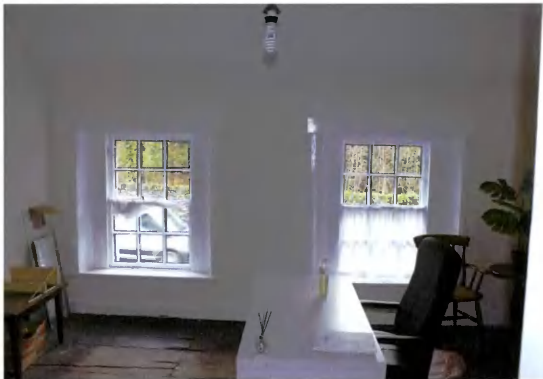
Figure 10: Two early 6/6-paned box sash windows on the first floor. (0660)
