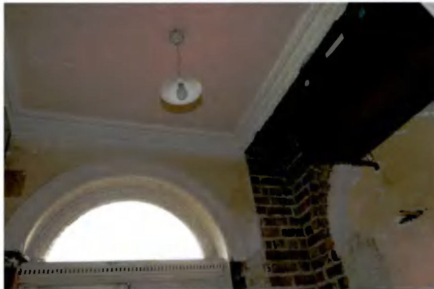
Plate 35: Ceiling in lobby
