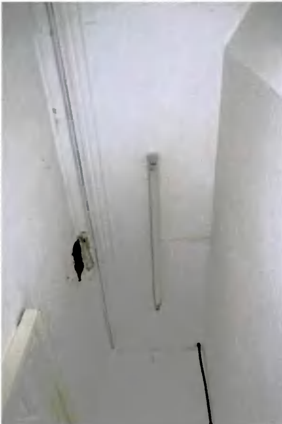
Plate 55: Ceiling in room F-13
