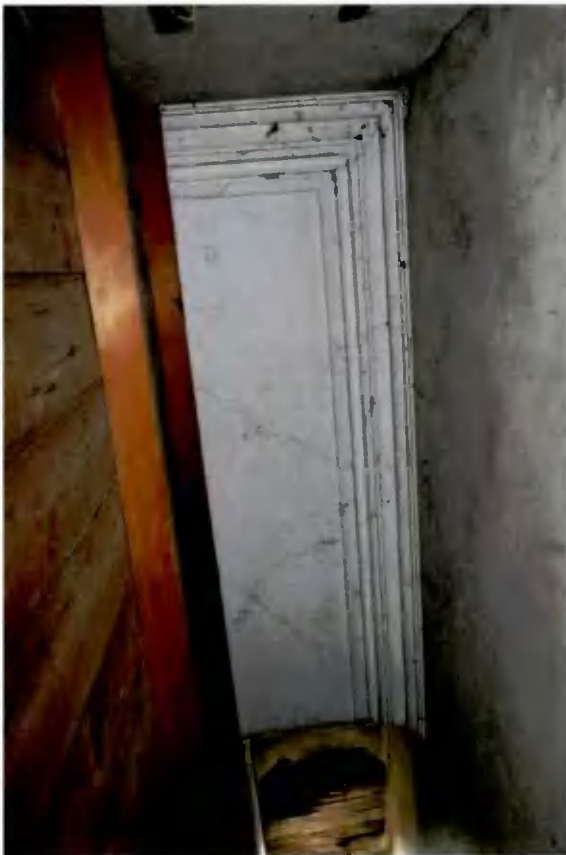
Plate 81: Cornice above staircase
