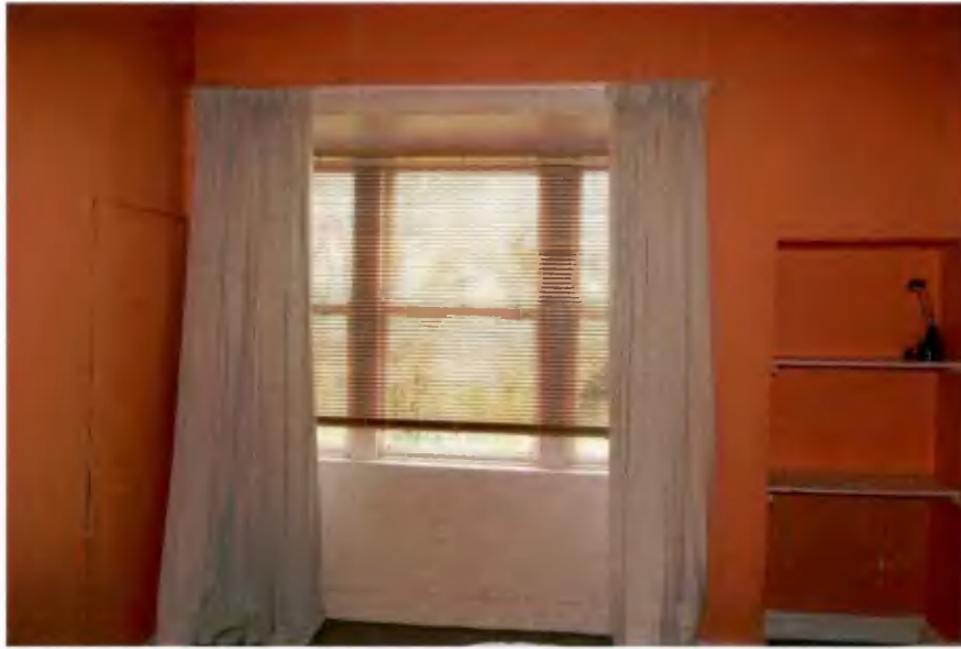
Plate 78: Window in northern wall of room S-8
