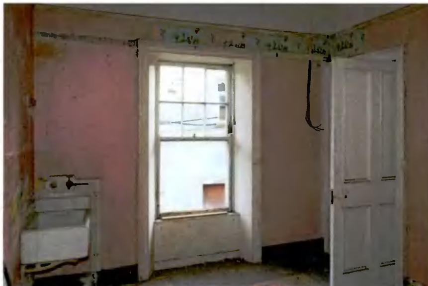
Plate 61: Southern wall of room F-16
