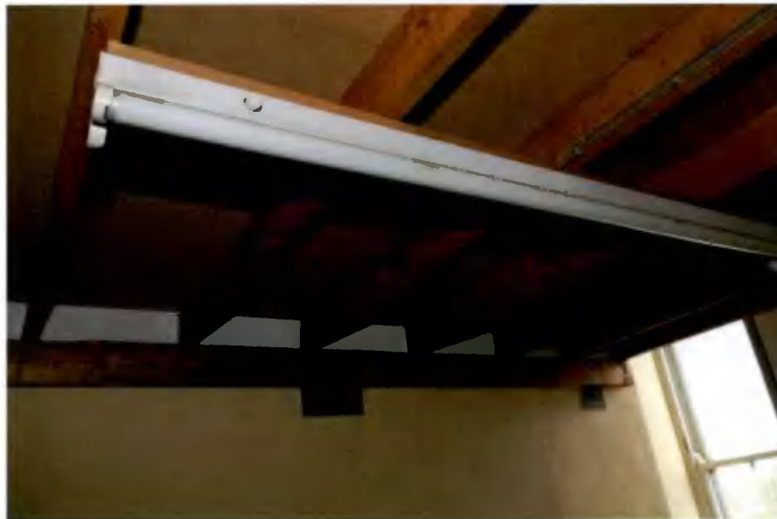
Plate 51: Ceiling in room F-11
