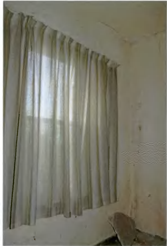
Plate 30: Window in room G-15
