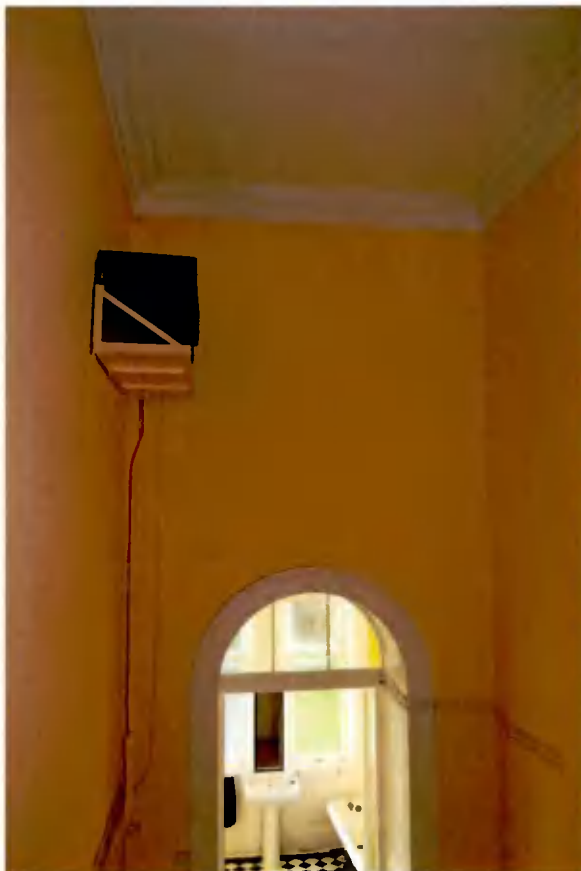
Plate 65: Ceiling over staircase
