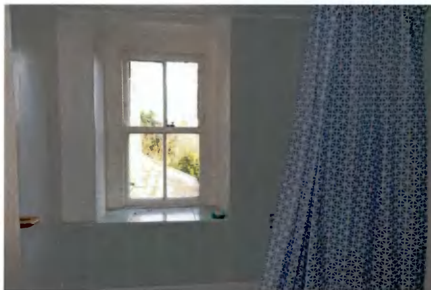
Plate 87: Window in eastern wall of bathroom
