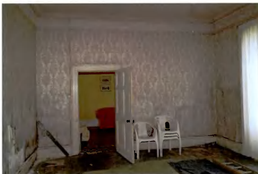
Plate 25: View to the west in room G-11
