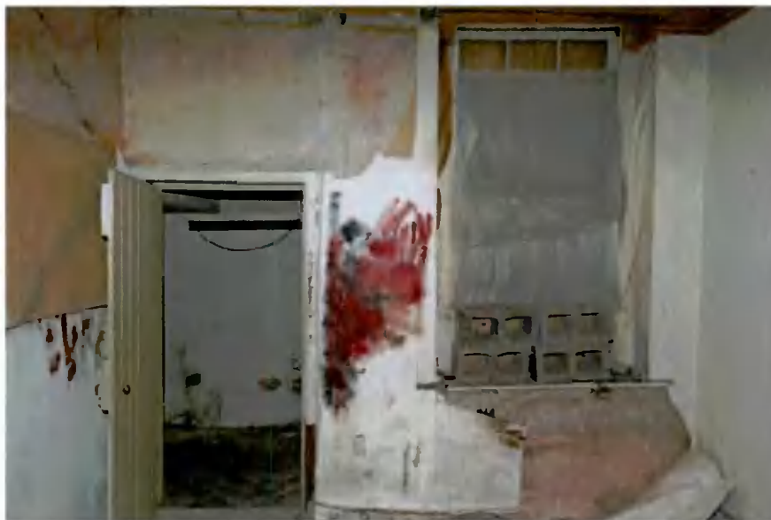
Plate 26: Door and window in room G-12
