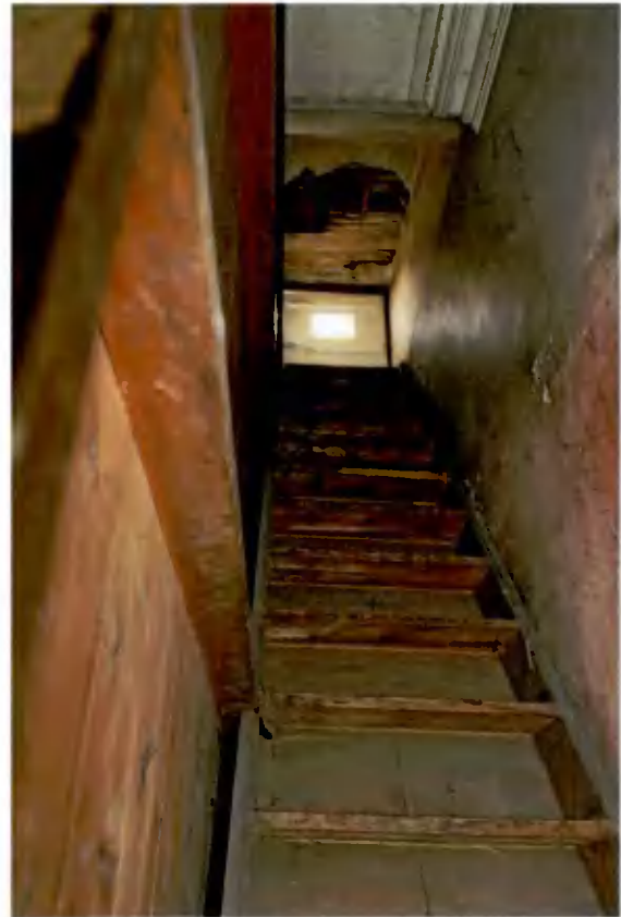
Plate 80: Stairs to attic
