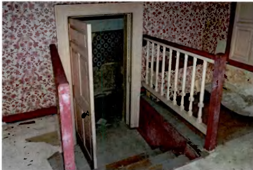
Plate 23: Steps leading to upper level of room G-10
