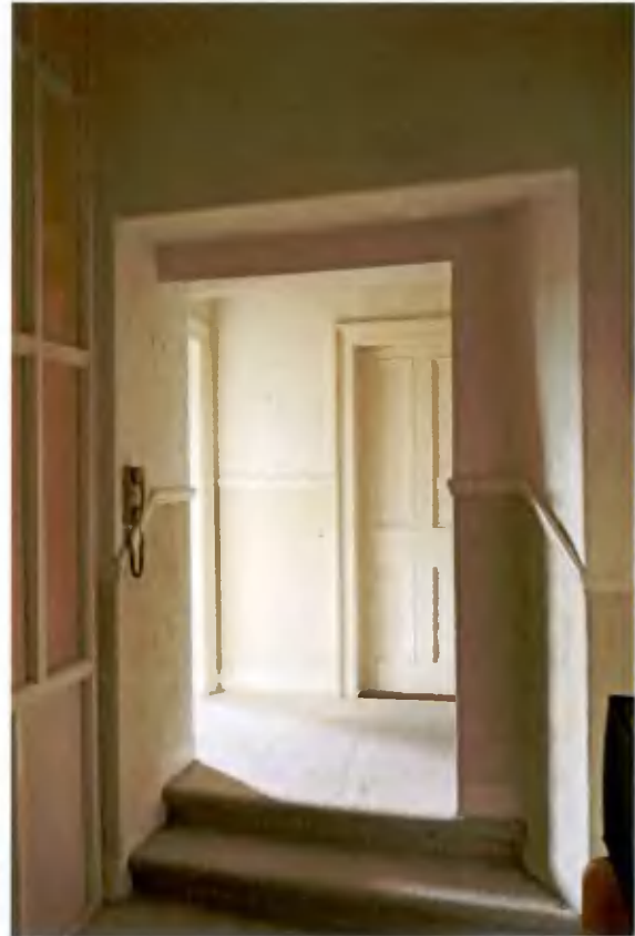
Plate 68: View to the west from lobby
