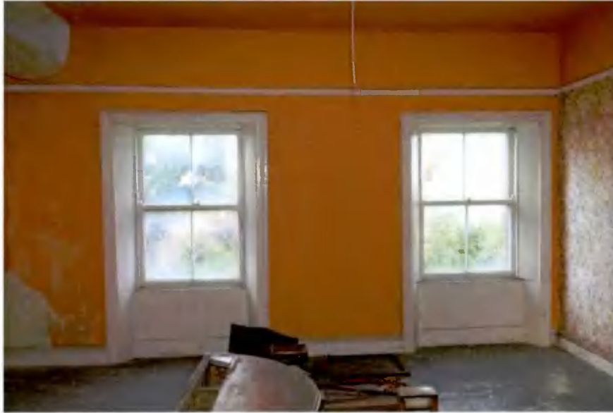
Plate 58: Northern wall of room F-15
