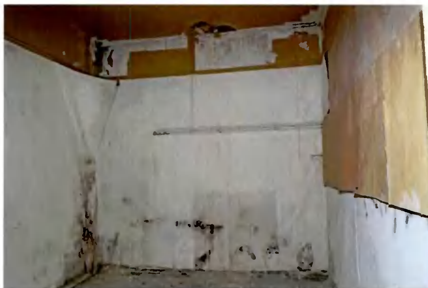
Plate 27: Western wall of room G-12
