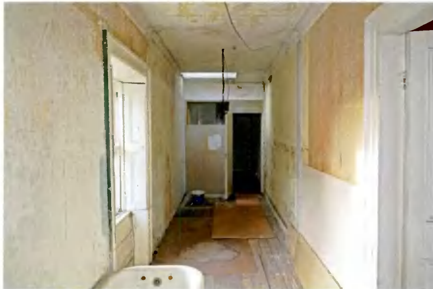
Plate 57: View westward along the corridor
