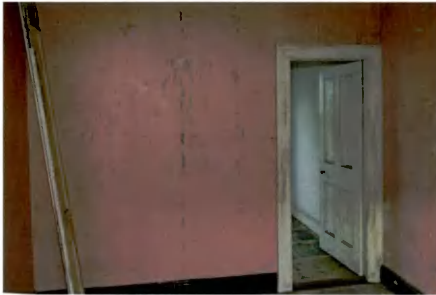
Plate 60: Northern wall of room F-16
