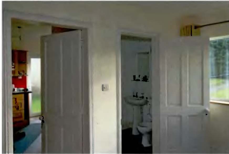
Plate 44: Eastern wall of room F-7
