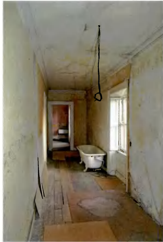
Plate 56: View eastward along the corridor
