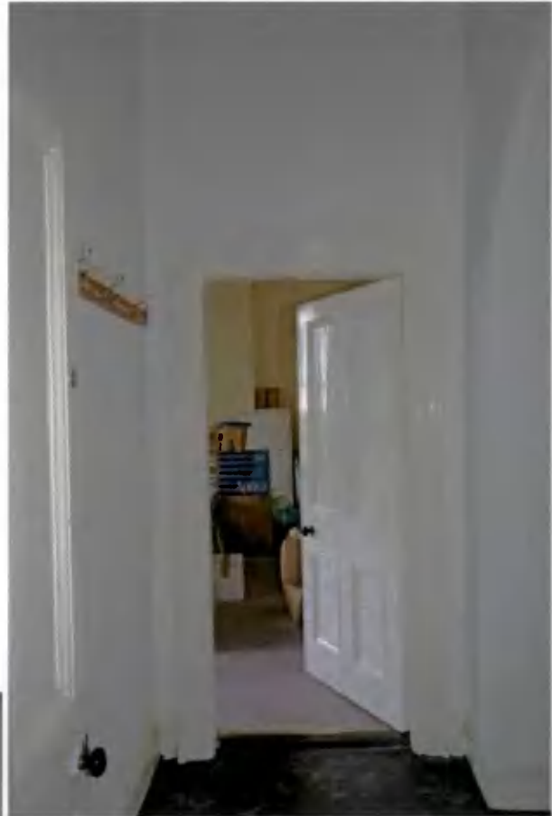
Plate 46: View eastward in room F-9 to door of room F-10
