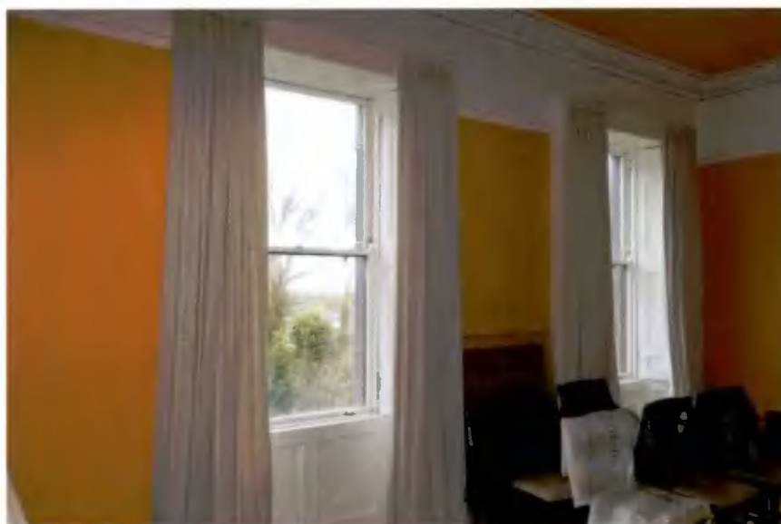
Plate 39: Windows in room F-4
