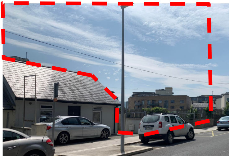
FIG. 43C: THE SITING, HEIGHT, SCALE, BULK AND DESIGN OF BLOCK B (&C) RELATIVE TO NOS. 8, 9 & 10
