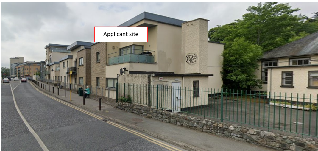
FIG. 6: VIEW SOUTH ALONG GREENHILLS RD WITH THE APPLICANT SITE ON THE RIGHT (GOOGLE EARTH PHOTOGRAPH)
