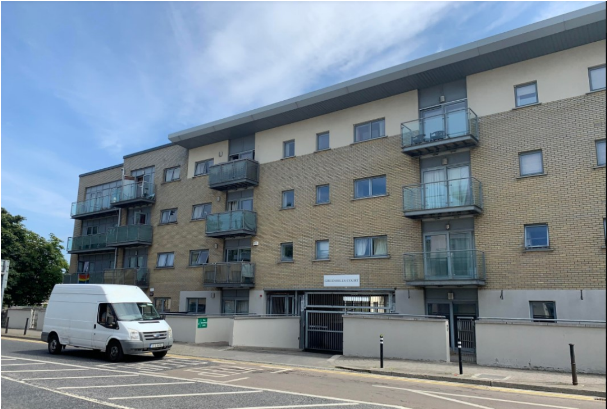
FIG. 5: 4 STOREY GREENHILLS COURT SCHEME ON THE EAST SIDE OF GREENHILLS ROAD APPEARS VISUALLY DOMINANT
