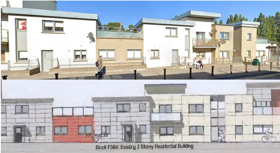
FIG. 9: 1 AND 2 STOREY PARTS OF THE EXISTING GREENHILLS COURT SCHEME
