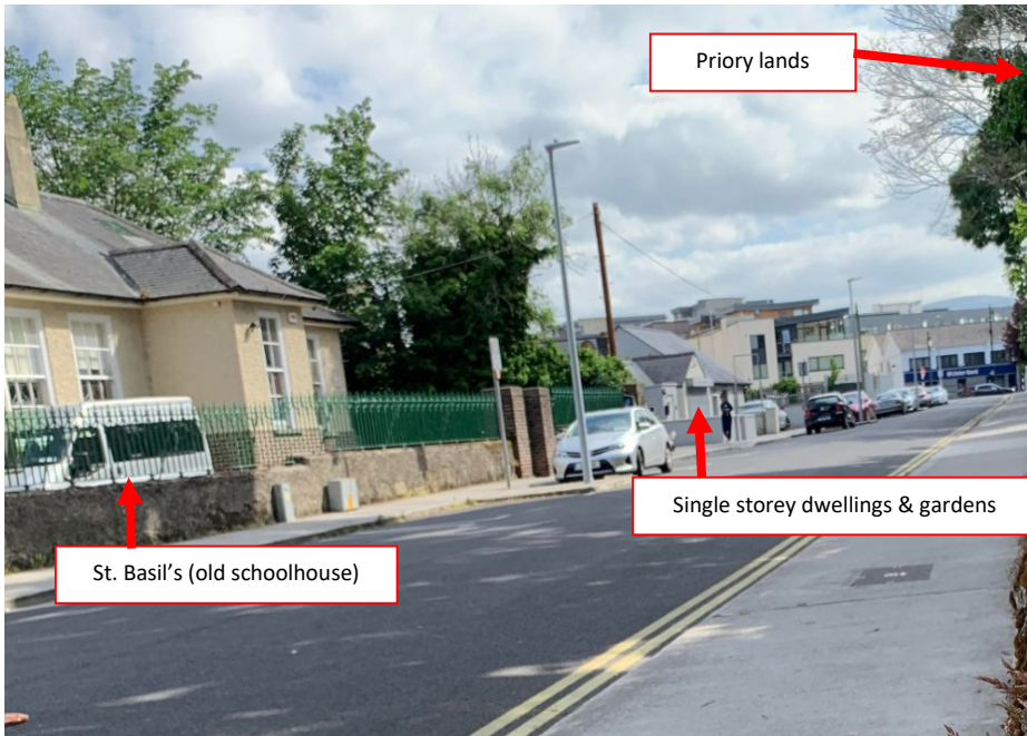
FIG. 3A: APPLICANT SITE CONTEXT TO OLD GREENHILLS ROAD – SINGLE STOREY ONLY ADJOINING APPLICANT SITE
