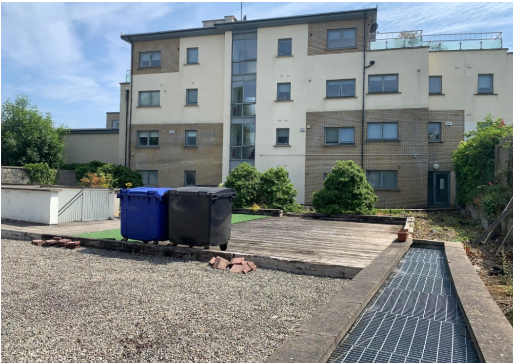
FIG. 4: EXISTING APPEARANCE OF GREENHILLS COURT'S OPEN SPACE AREA (& PROPOSED CENTRAL OPEN SPACE AREA) – 2
