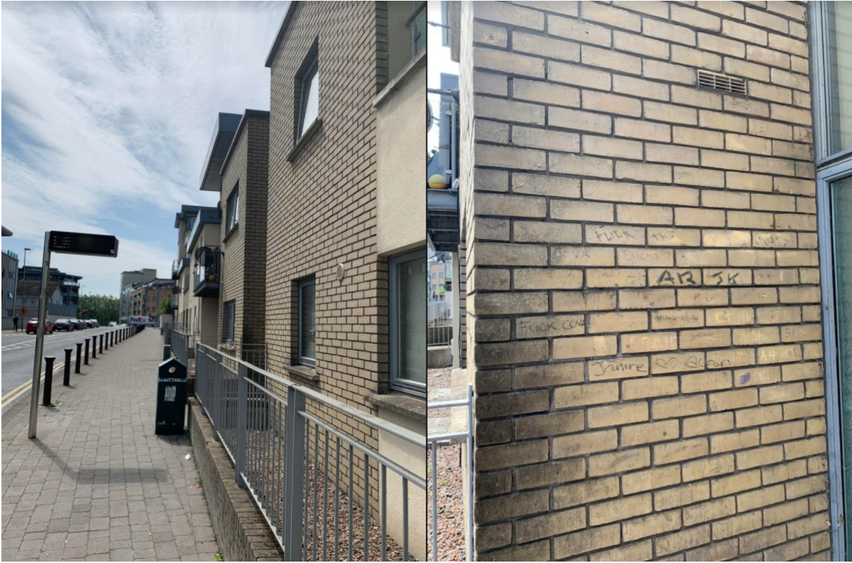
FIG. 1: POOR STREETScape INTEGRATION, ELEVATION LOCATED CLOSE TO FOOTPATH, NO PLANTING, POOR MAINTENANCE, ETC.
