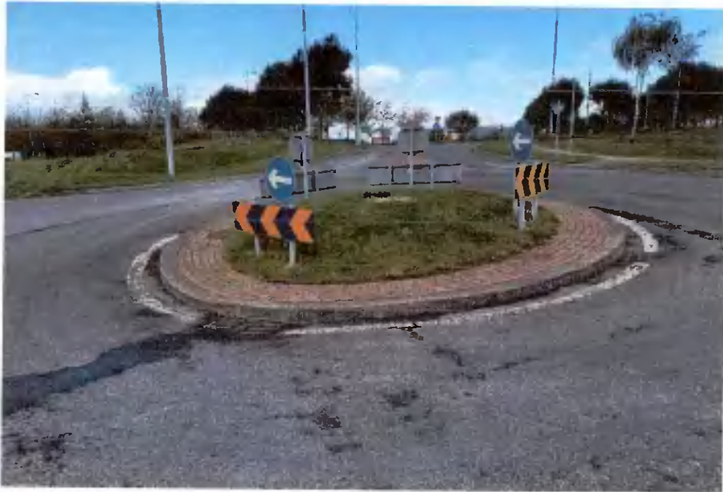
Figure 2.3: Roundabout on Brownsbarn access looking towards Roundabout 2 (source: SRC, May 2021)
