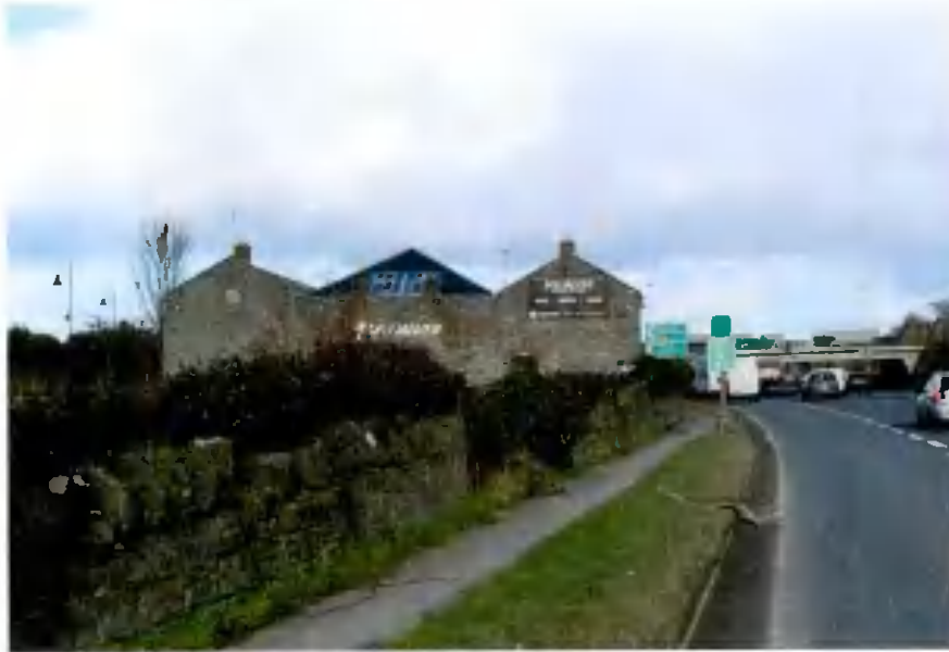
Plate 7: View of stables from approximately 80 metres to the west
