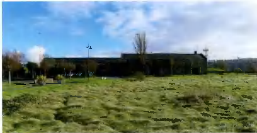
Plate 1: Royal Garter Stables, seen from the application site
