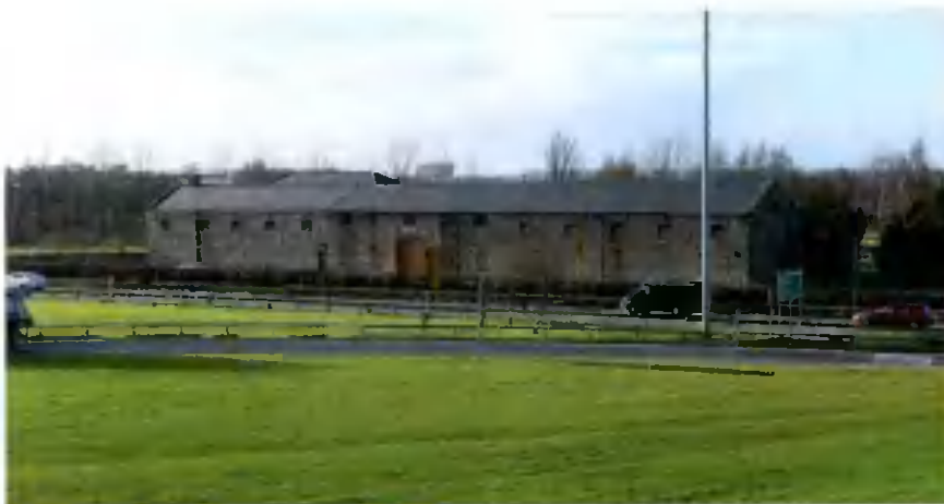
Plate 2: Royal Garter Stables, seen from the south, across the Naas Road
