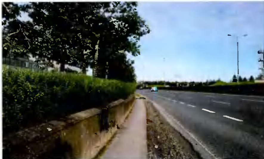
Plate 9: Montage view from approach on northbound side of Naas Road
