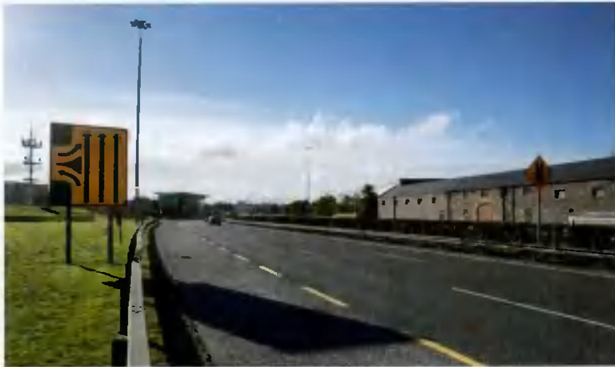
Plate 10: Montage view of development from southern side of Naas Road
