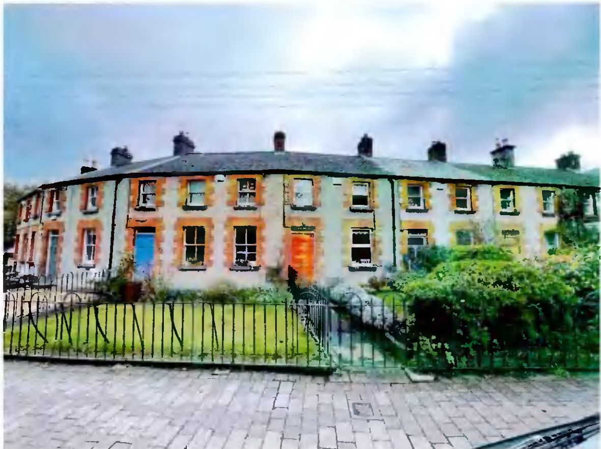
Photo of the Terrace as viewed from the Public Footpath
