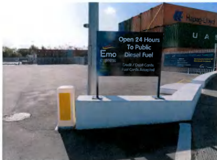
Figure 7: Boundary wall and signage to Crag Avenue (front boundary)
