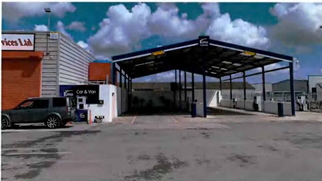
Figure 4: Truck fueling area and Canopy
