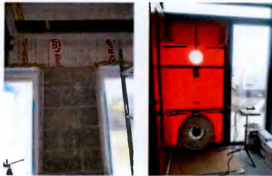
Figure 3 – Air Tightness Testing
