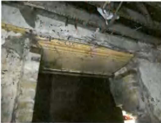
Figure 33: Timber lining to window in room G03
