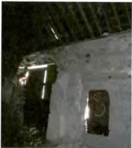
Figure 25: Missing lintel and weakened timber lintels above openings on north elevation
