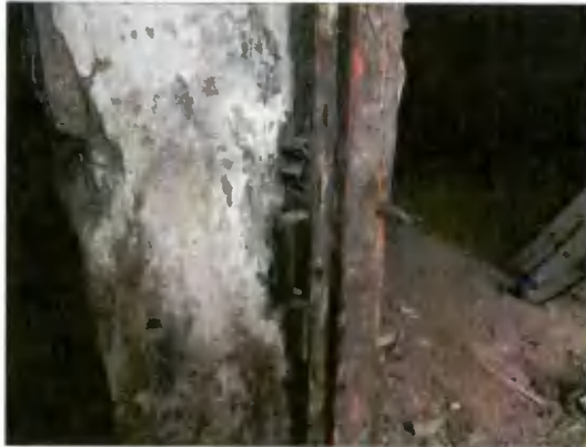
Figure 31: Door frame in room G01
