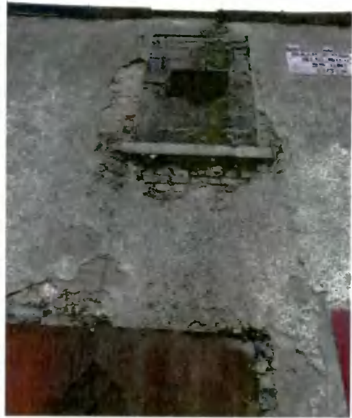
Figure 24: Detail of west elevation
