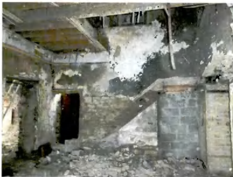
Figure 39: Wall marking of dog-leg stairs in hall (room G03)
