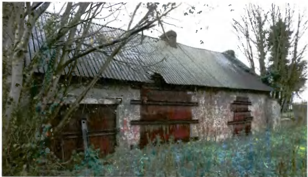
Figure 20: South elevation of single-storey section
