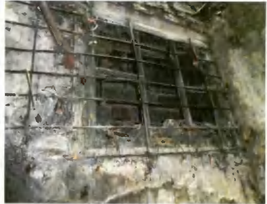
Figure 32: Timber casement window in room G01
