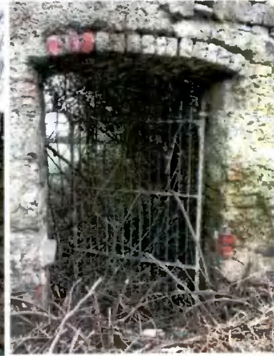
Figure 43: Gate in walled garden wall
