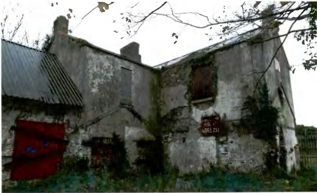
Figure 21: East and north elevations of two-storey section
