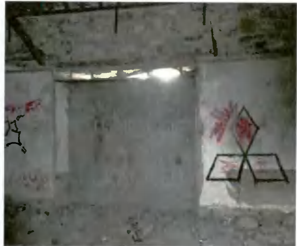
Figure 25: Missing lintel and weakened timber lintels above openings on north elevation
