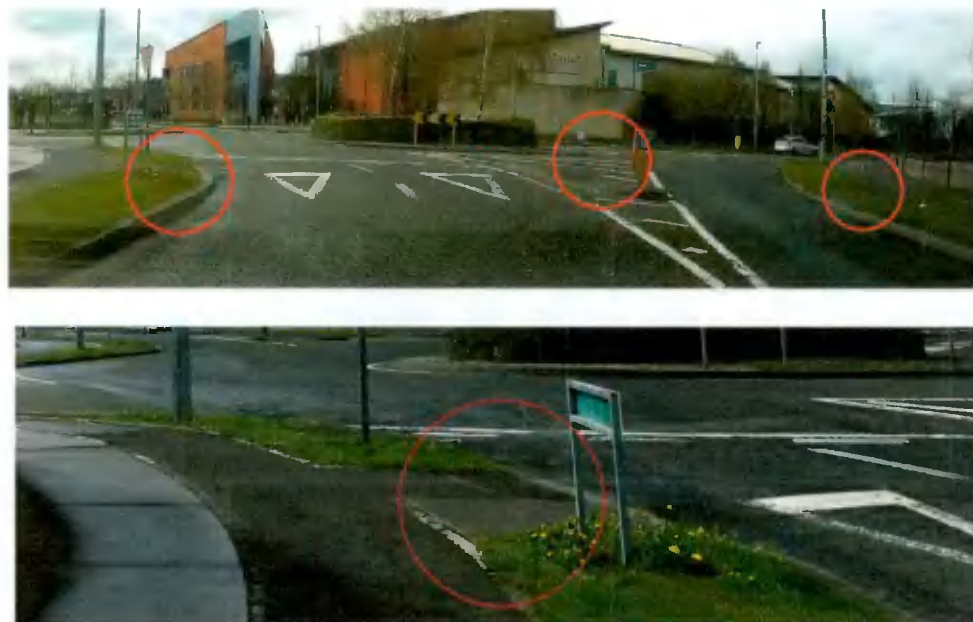
Figure 8 Griffeen Av roundabout at school entrance – poor pedestrian facilities
