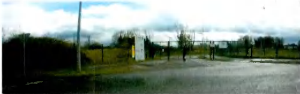
Figure 2 – Main access to school off a roundabout on Griffeen Avenue
