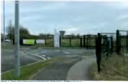
Photo 1 - View of Existing entrance to Primary School from Griffeen Avenue
