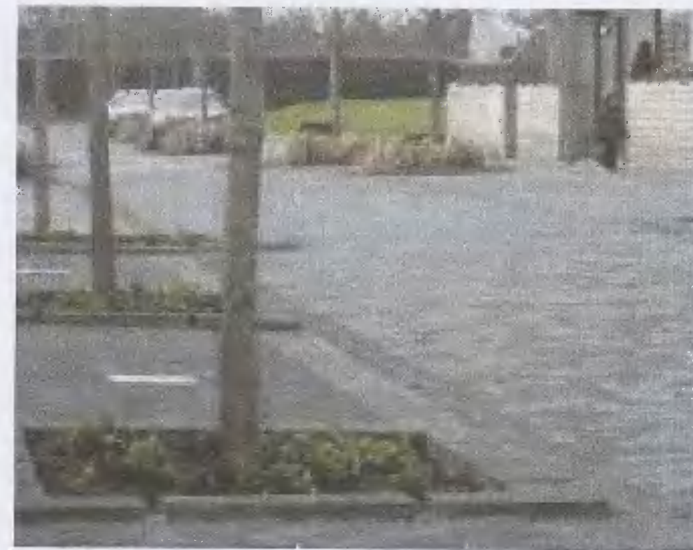
FIGURE 19.16: EXAMPLE OF INLETS TO ALLOW SURFACE WATER RUNOFF TO INFILTRATE INTO TREE PITS. TAKEN FROM CIRIA REPORT C753 THE SUDS MANUAL.
