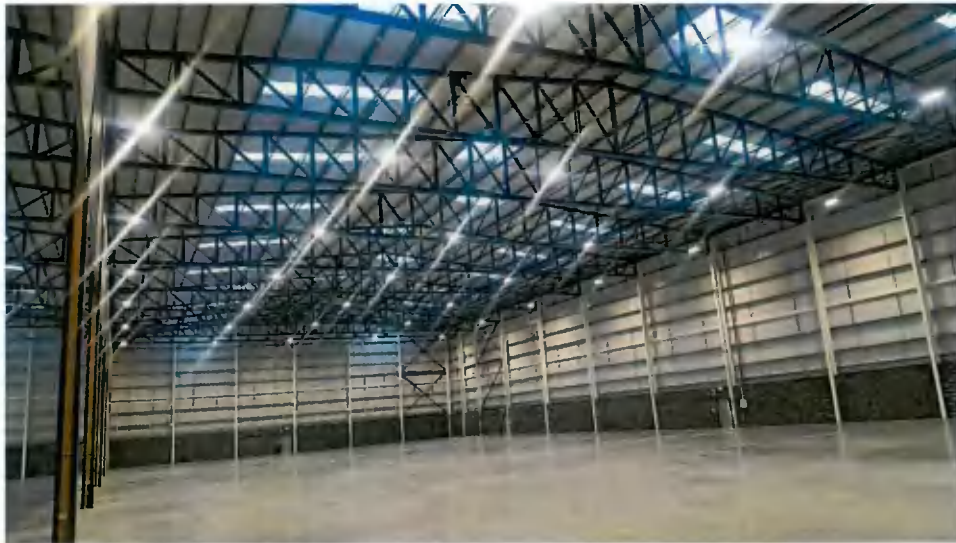
Typical clear open space warehousing facility
