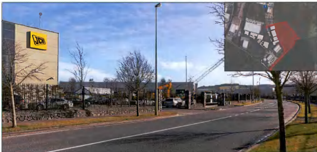
Figure 5.3: Proposed Image of the Subject Lands when Viewed from Jordanstown Road looking South with an Insert Showing the location of the Viewpoint.
