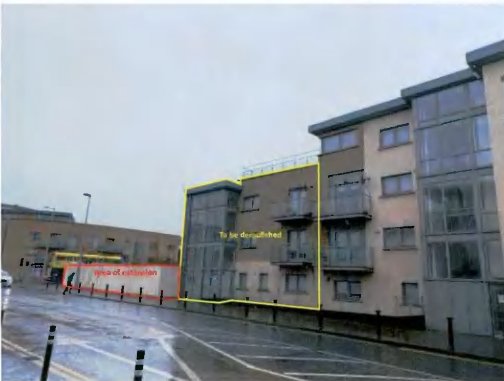
Plate 3. South end of development showing porting to be demolished and area of extension
