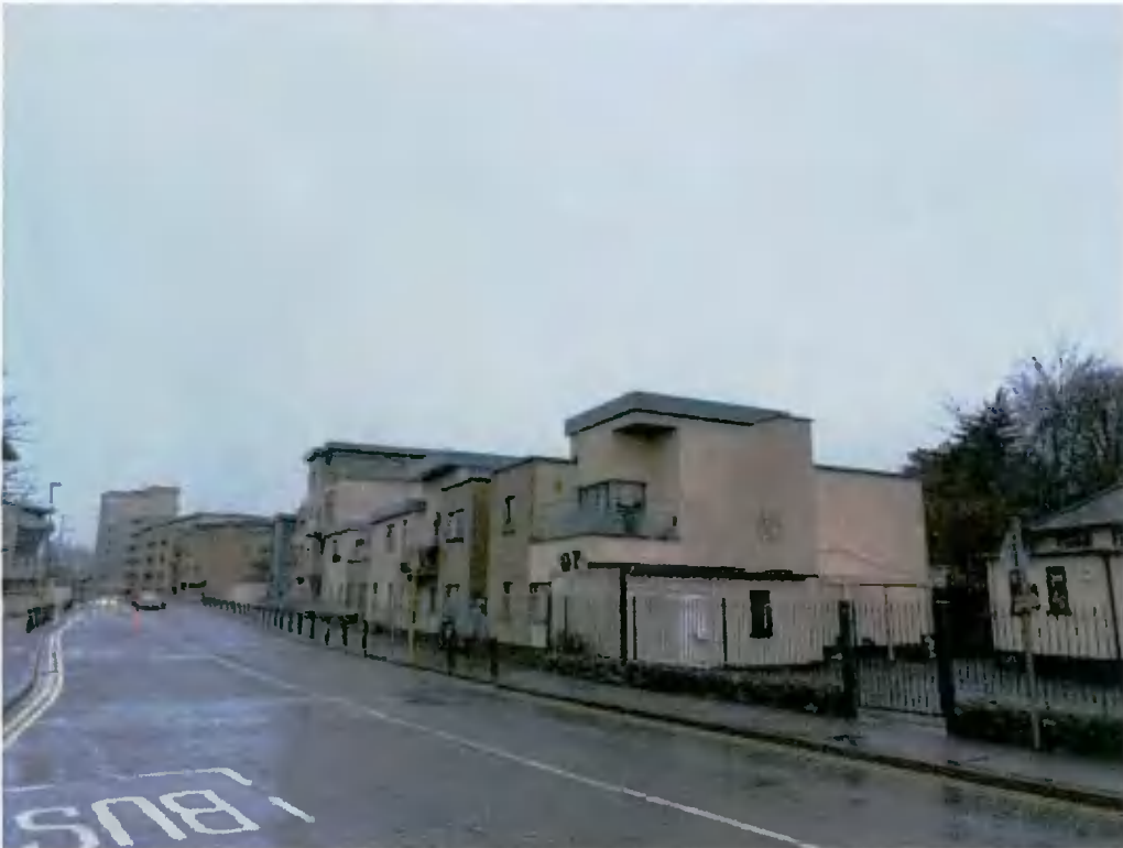
Plate 2 Existing development from the north, to be retained
