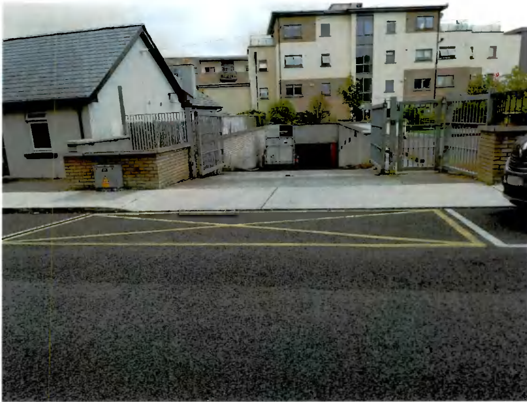
Image 3: Existing Basement Access
