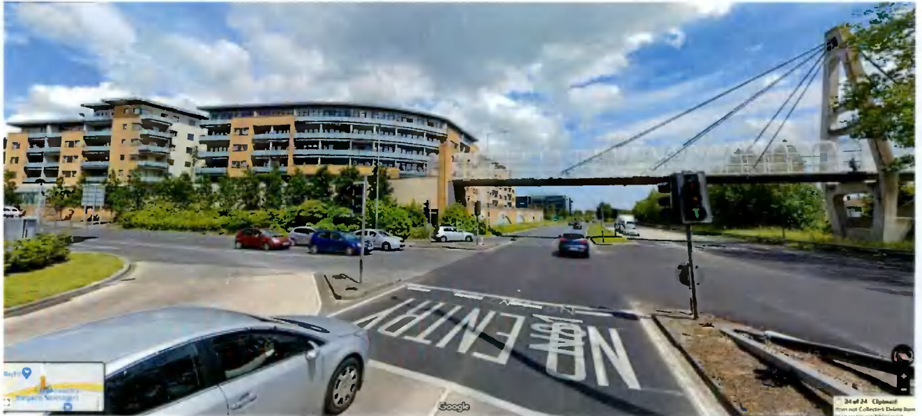
Figure 3-6: Tallaght Bypass looking north-east ( Tallaght Bypass @Googlemaps )
