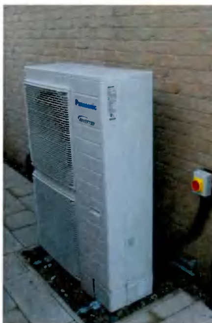
Fig. 4.4 – Typical Air Source Heat Pump Installation
