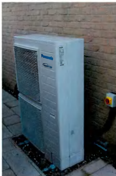
Fig. 4.4 – Typical Air Source Heat Pump Installation
