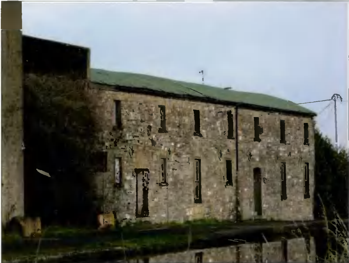
Figure 17 Two-storey former mill building (RPS ref. no. 118 / NIAH ref. no. 1120405).
