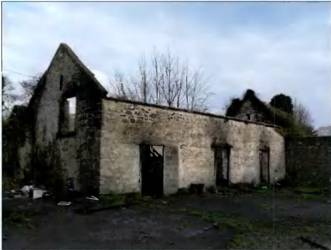
Figure 15 Nineteenth century farm building, located to north-west corner of Field 6.
