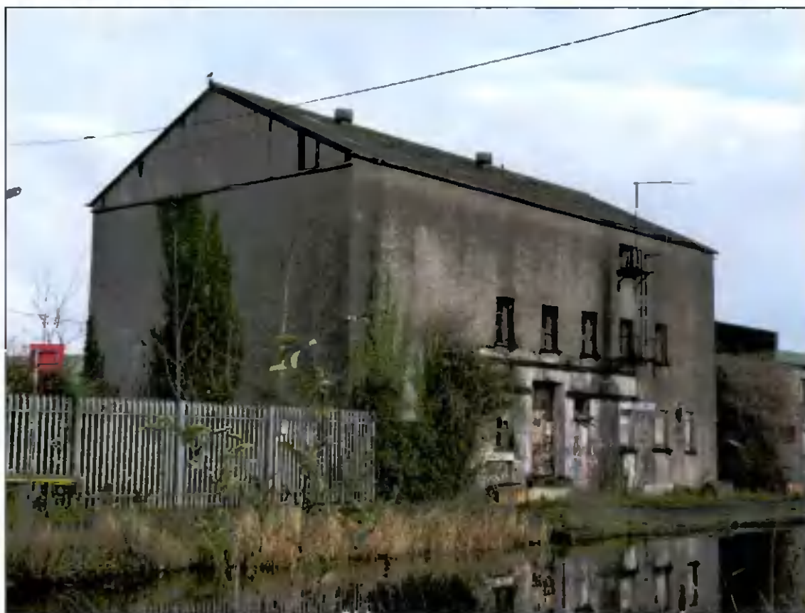
Figure 19 Former mill building (NIAH ref. no. 11204055).
