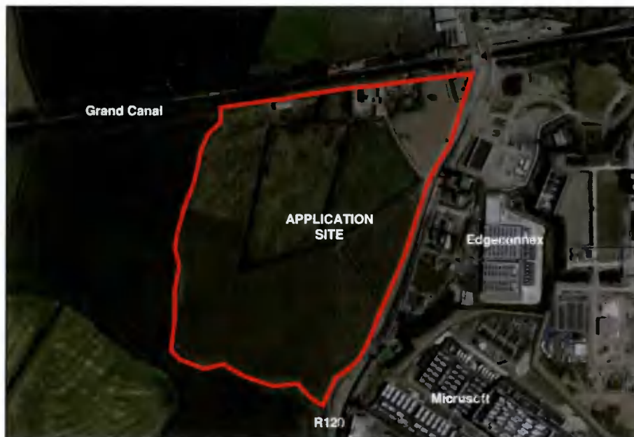
Figure 2.1 Aerial view of application site (refer to architectural drawings of Existing Site Plan and all buildings to be demolished that accompany the application for greater detail)
