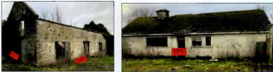
Figure 5.1 Derelict and abandoned residential properties within northern RU zone to be demolished under the application
