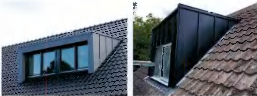
Reference pictures of a dormer finished in natural grey colour zinc (left) and anthracite zinc (right).
