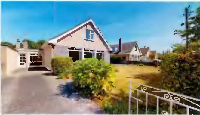
Picture of the existing house seen from the road (south-west)
