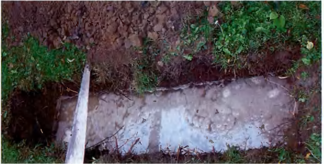
Pit during test
