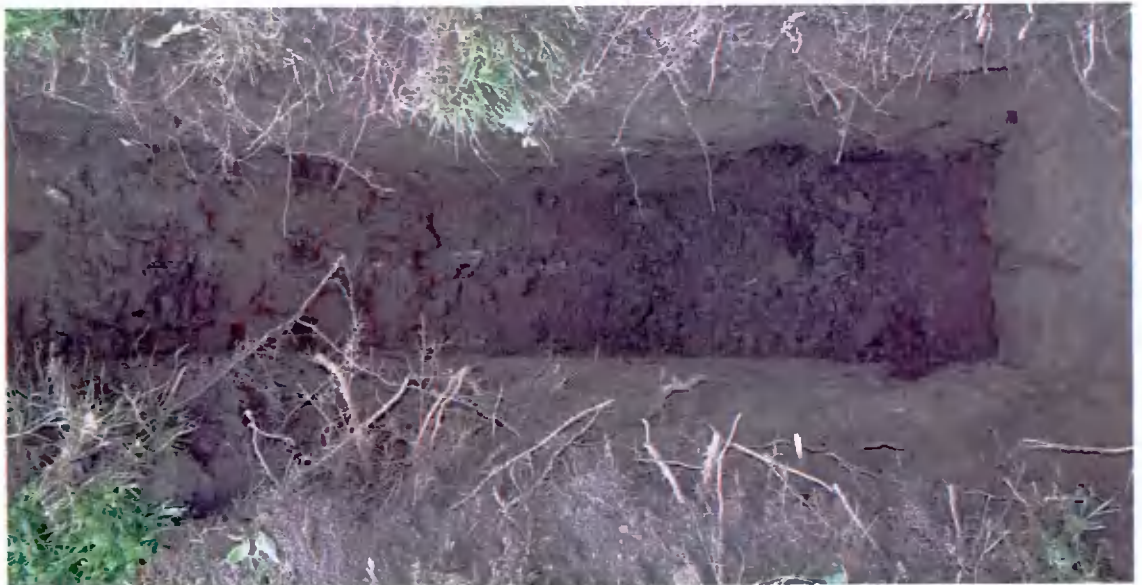
Test Pit before water added – Depth 1.5m
